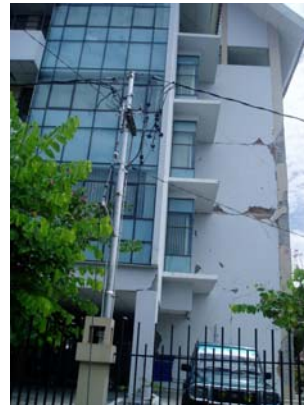
BPKP building, Padang, West-Sumatra
