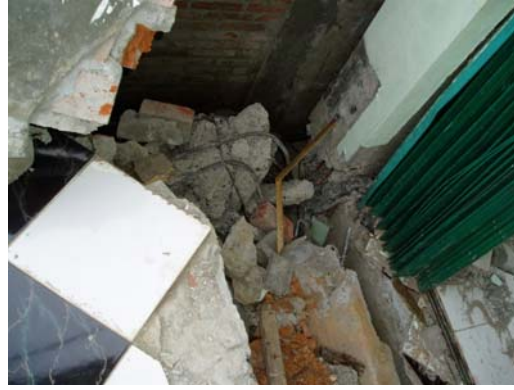
Figure 19. (Cont'd): Collapsed of “first soft story” building at Padang Jati Rd., Tanah Patah, Bengkulu
