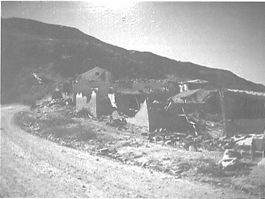
Figure 2 – A high percentage of the adobe buildings was damaged.
