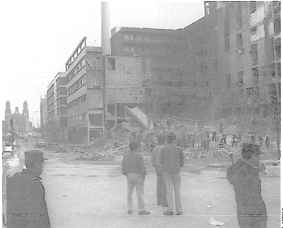
Collapsed St. Regis Hotel
