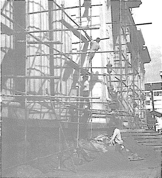
(Above) Six workmen sealed crack surfaces with a temporary seal and two technicians manned each of seven pumping machines. (Below) Repaired roof structure shows typical concrete cracking pattern.
