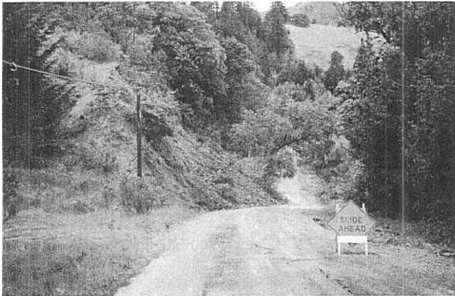
Landslide on the Mattole Road between Petrolia and Ferndale caused tree to fall on overhead lines
