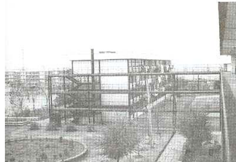
FIGURE 1A: Typical Building: Poblacion Republica popular China, located in Vina del Mar, an area affected by the March 3, 1985 earthquake. These buildings suffered no damage.
