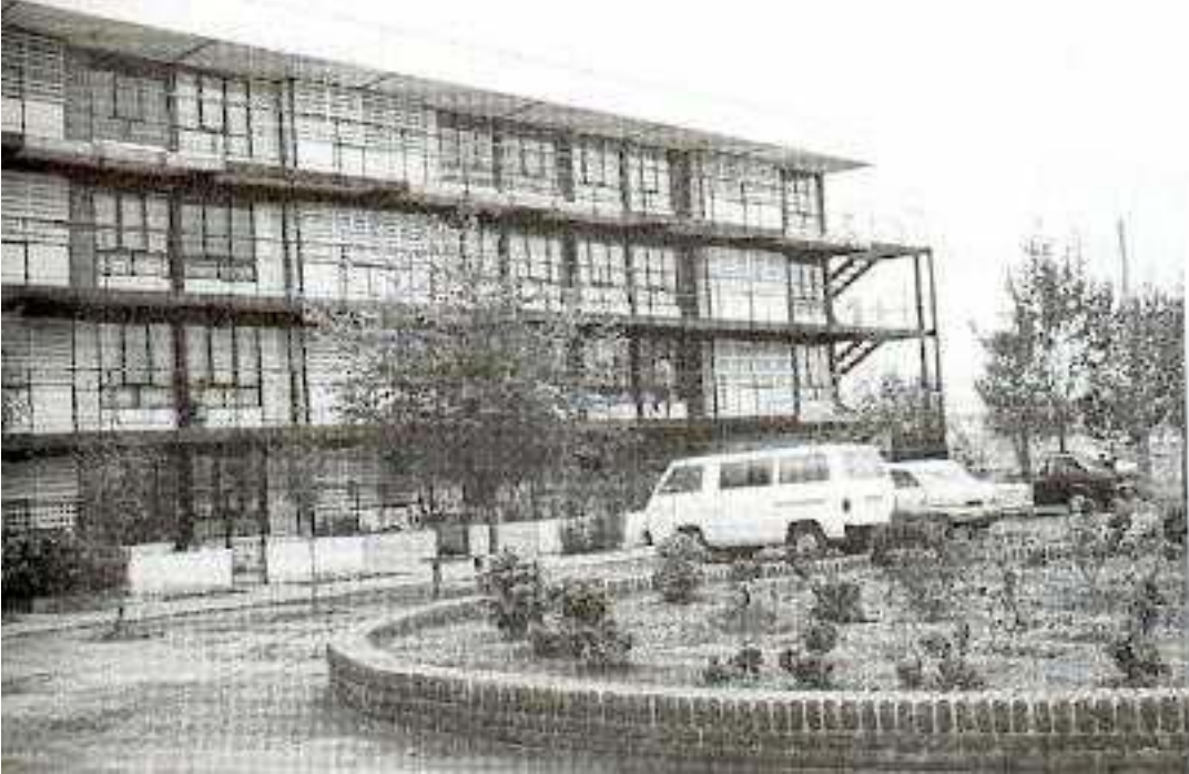
FIGURE 1B: Typical Building: Poblacion Republica popular China, located in Vina del Mar, an area affected by the March 3, 1985 earthquake. These buildings suffered no damage.
