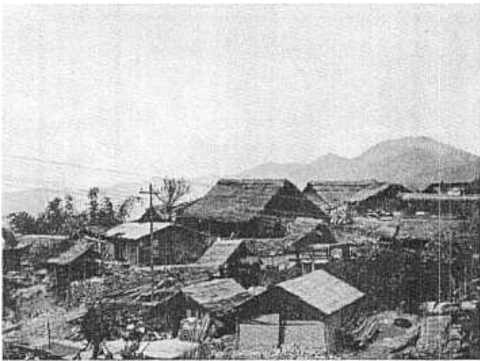
Photo 1. Yansoi Village houses, after earthquake shaking of intensity 9.
