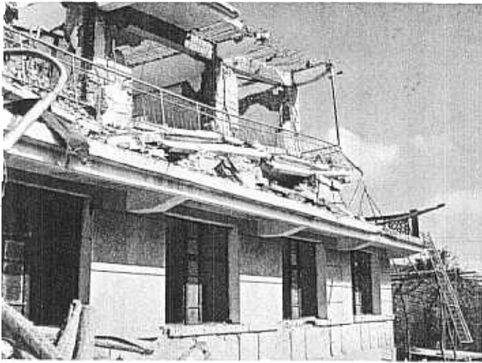
Photo 5. Administrative building, Yansoi Village, intensity 9. Two-storied reinforced concrete structure.
