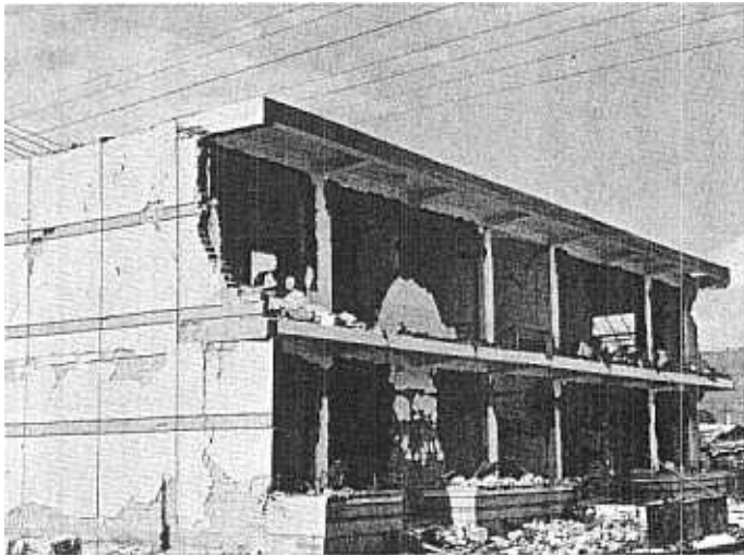
Photo 3. Mengerseng tea factory, after earthquake shaking of intensity 9. Masonry structure with hollow block walls and cast-in-situ reinforced concrete floors.
