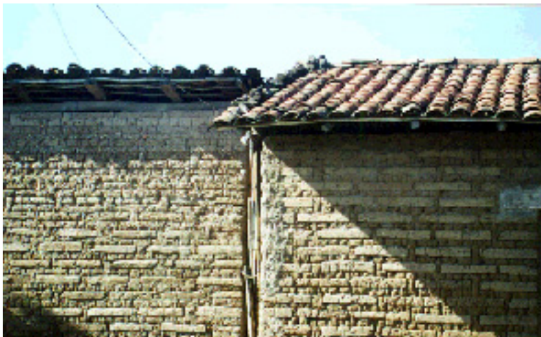
FIGURE 4A: Critical Structural Details-An illustration of wood beams supporting clay tiles and roof-walls connections
