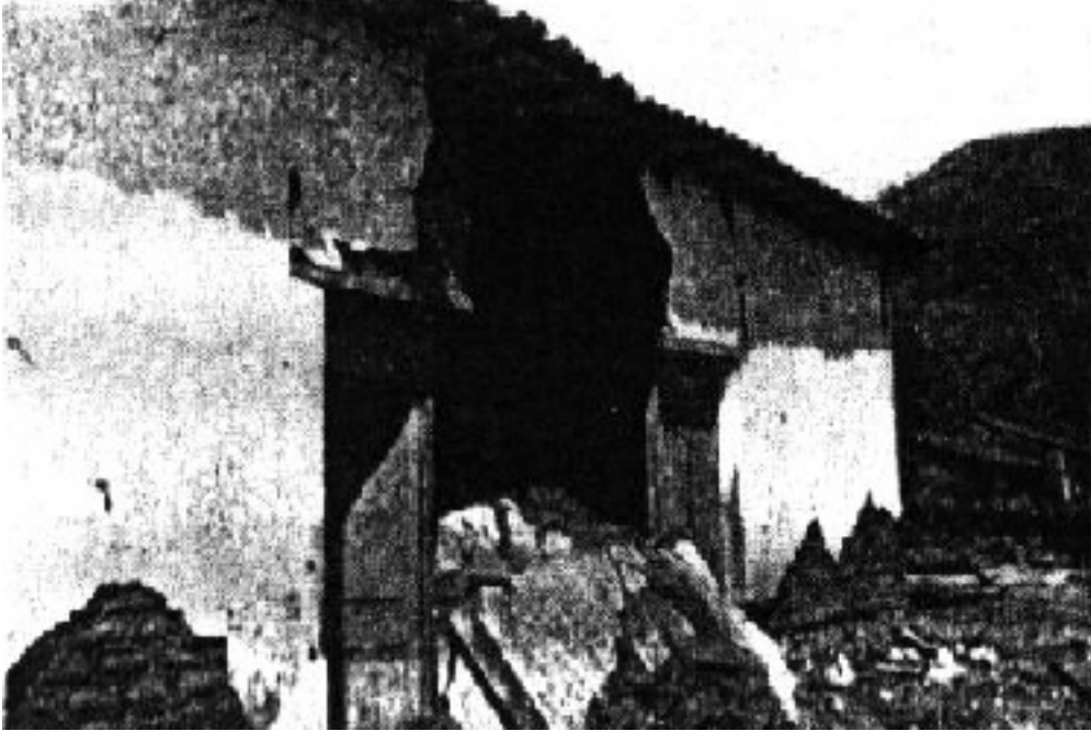
FIGURE 6A: Damage to an adobe house in the 1936 San Vicente earthquake
