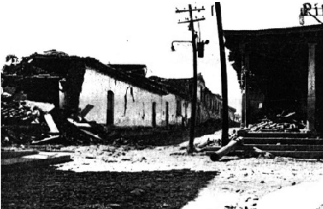
FIGURE 6B: Damage to adobe houses in the 1936 San Vicente earthquake
