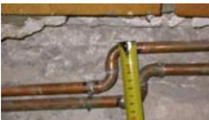
Figure 14. Plan view of two adjacent buildings with a common pipeline system that had a differential settlement of about 5 cm (ITSAK team). (Photo taken after repairing.)
