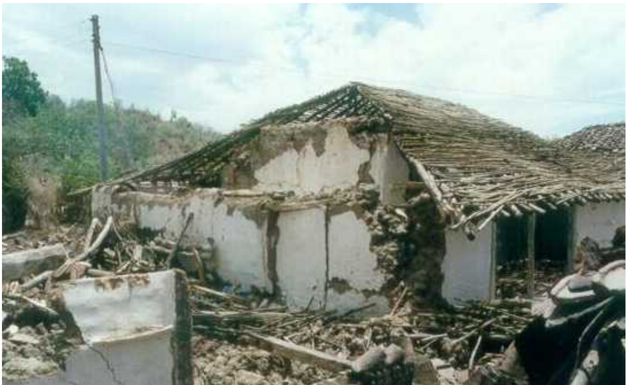
FIGURE 6A: Typical Earthquake Damage - Cracking and Separation of Walls in the 1997 Jabalpur earthquake (Source: Sudhir K. Jain, IIT Kanpur)
