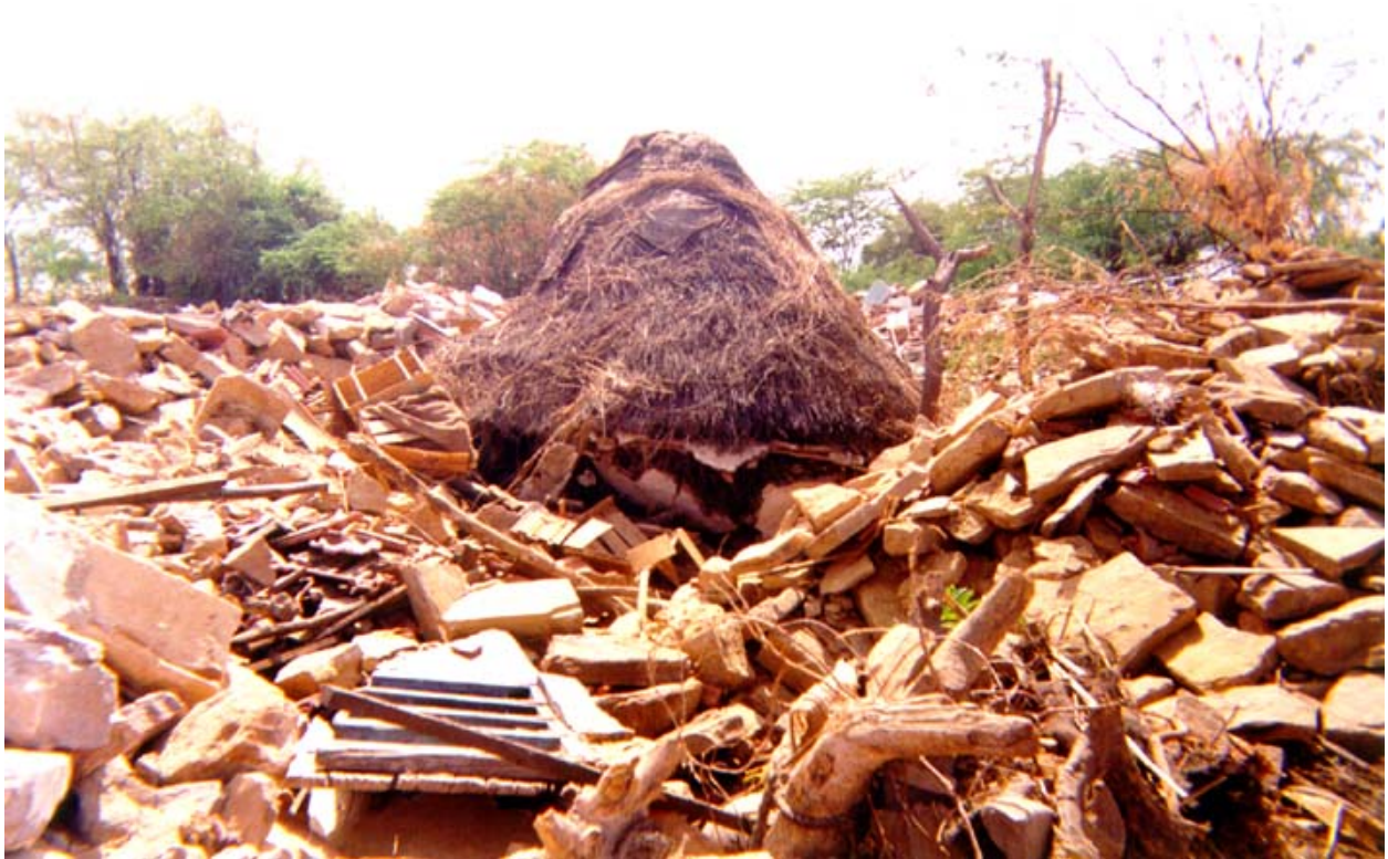
Figure 6B: A Photograph Illustrating Typical Earthquake Damage (2001 Bhuj earthquake)
