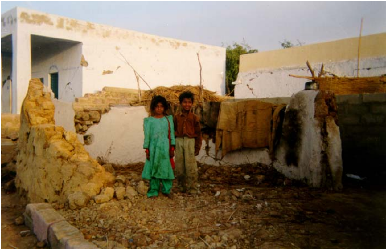
FIGURE 6A: A Photograph Illustrating Typical Earthquake Damage (2001 Bhuj earthquake)
