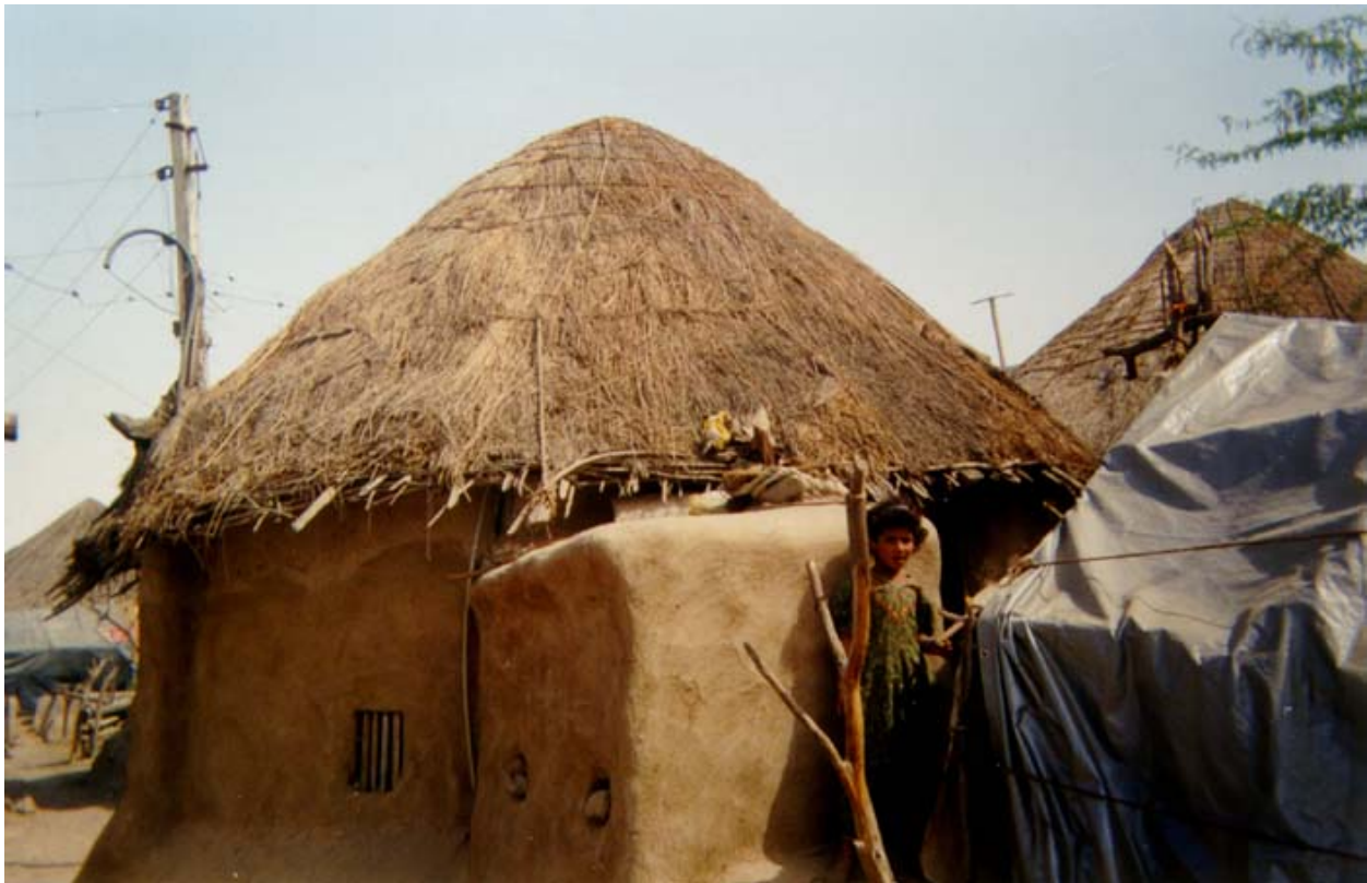
Figure 1D: Typical Building
