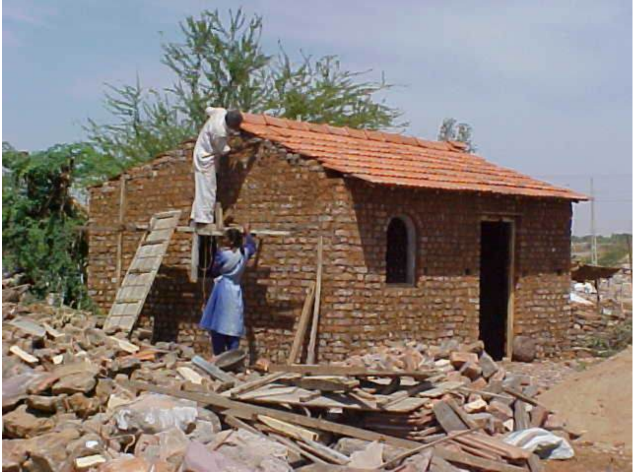
FIGURE 2C: Key Loadbearing Elements - Laying of Mangalore Roof Tiles (Source: Sudhir K. Jain, IIT Kanpur)
