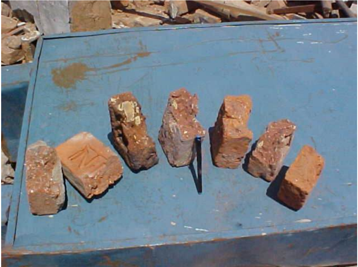
FIGURE 5B: Construction Deficiency - Poor Quality Bricks (Source: Sudhir K. Jain, IIT Kanpur)
