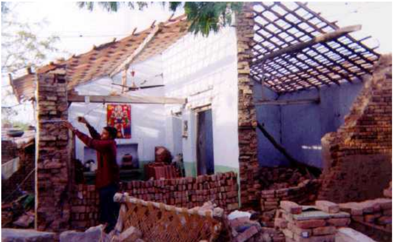
FIGURE 2A: Key Load-bearing Elements - typical village house in Gujarat (Source: IIT Powai 2001)
