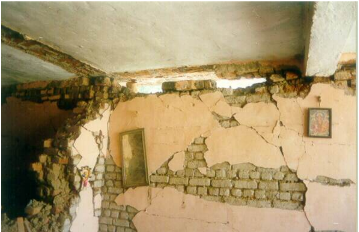
FIGURE 6A: Typical Earthquake Damage - Failure of Unreinforced Masonry Walls in the 1997 Jabalpur Earthquake (Source: Sudhir K. Jain, IIT Kanpur)
