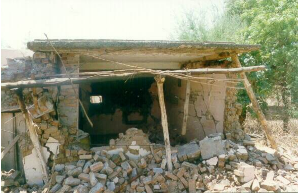
FIGURE 6A: Typical Earthquake Damage - Failure of Unreinforced Masonry Walls in the 1997 Jabalpur Earthquake (Source: Sudhir K. Jain, IIT Kanpur)
