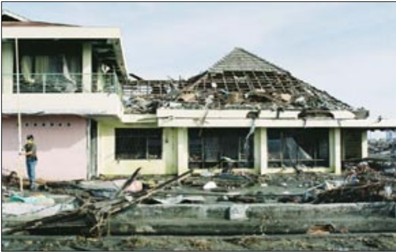
Figure 3. Roof tiles were removed by the flooding wave in Banda Aceh.
