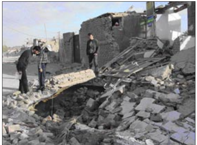
Figure 8 Qanat sink-hole that damaged a nearby structure (IIEES 2003).
