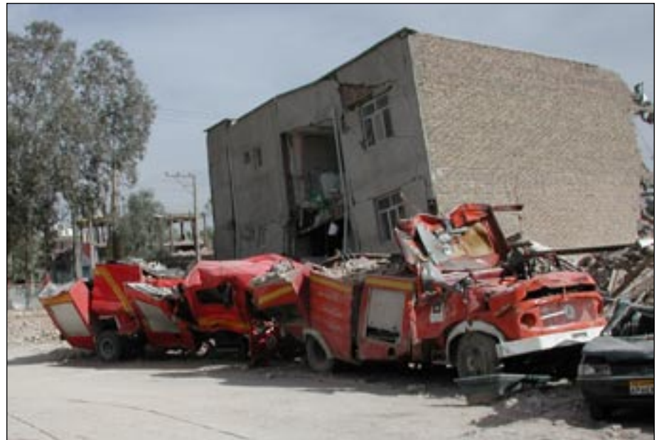
Figure 22 Fire engines were crushed under the collapsed fire station.
