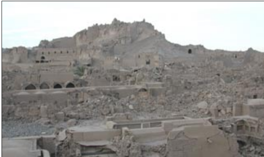
Figure 13 View of damage to the Arge-Bam historical citadel.
