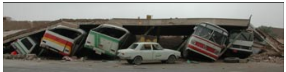
Figure 23 Collapse of the bus terminal roof trapped city buses.
