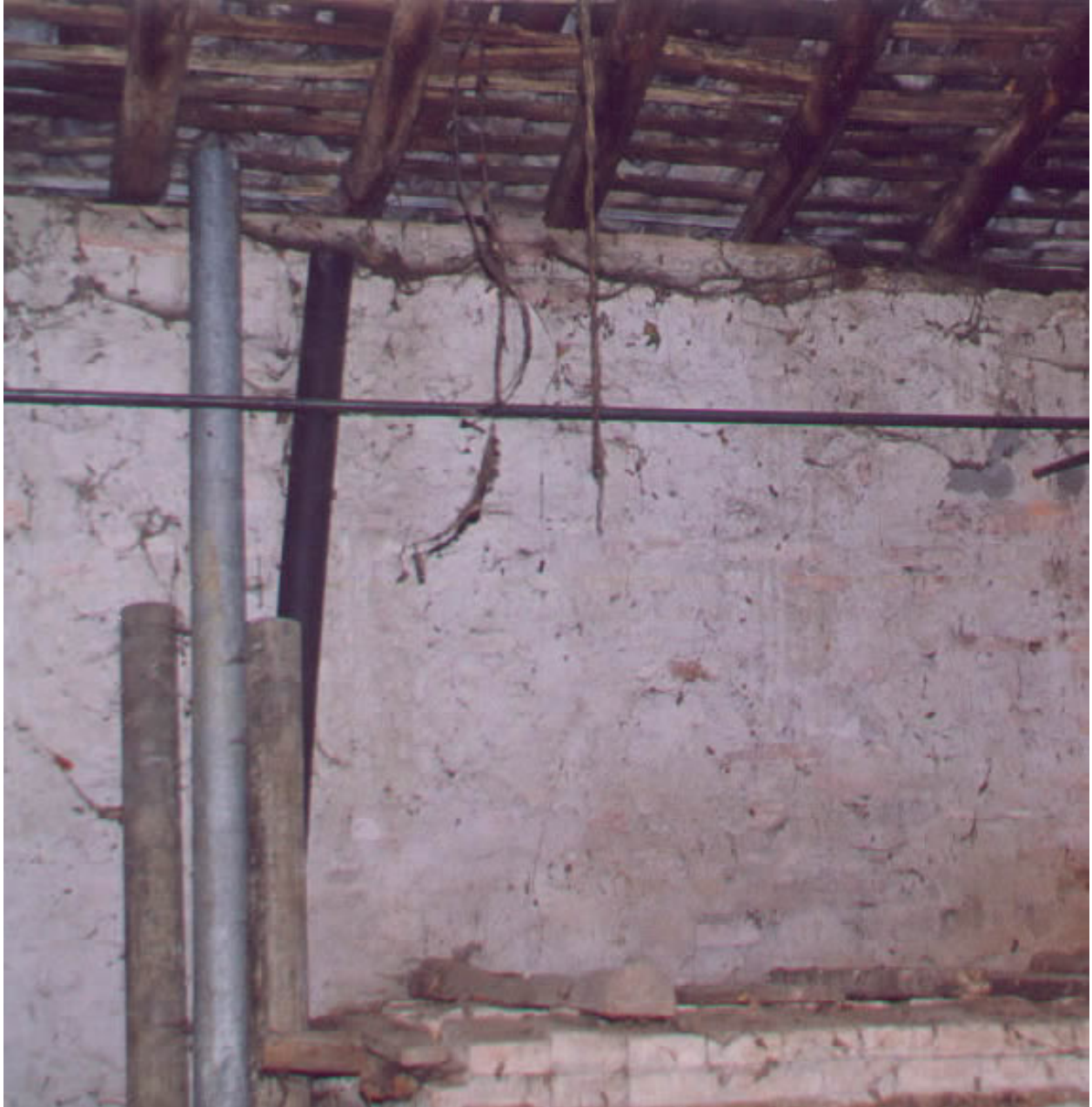
FIGURE 6B: Seismic strengthening technique - installation of the iron ties
