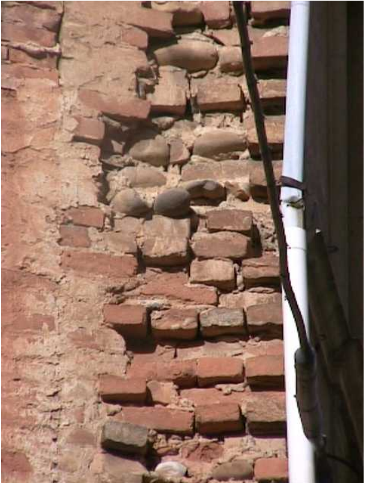
FIGURE 4B: Brick Walls Supporting the Cross-Vault System
