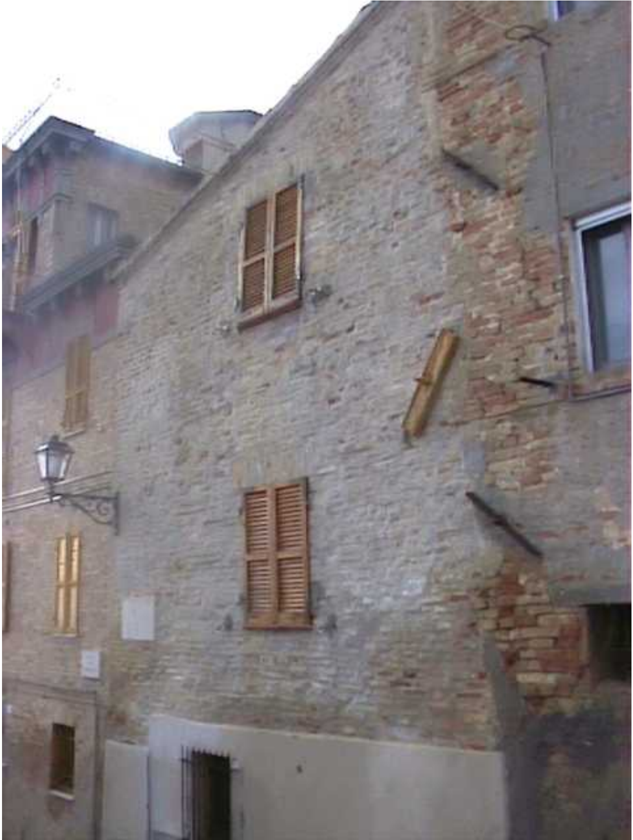
FIGURE 7A: Illustration of Seismic Strengthening Techniques
