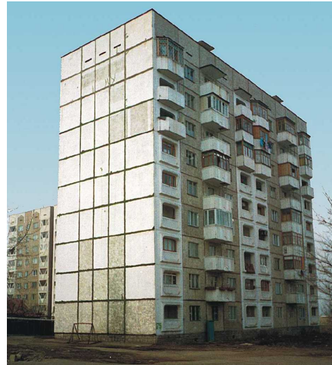
FIGURE 1A: Typical Building
