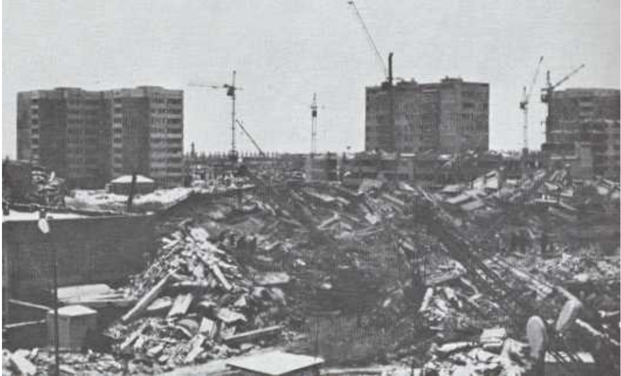
FIGURE 6: Earthquake Damage - Large Panel Buildings Remained Undamaged in the 1988 Spitak (Armenia) Earthquake (Source: EERI Armenia Earthquake Reconnaissance Report)
