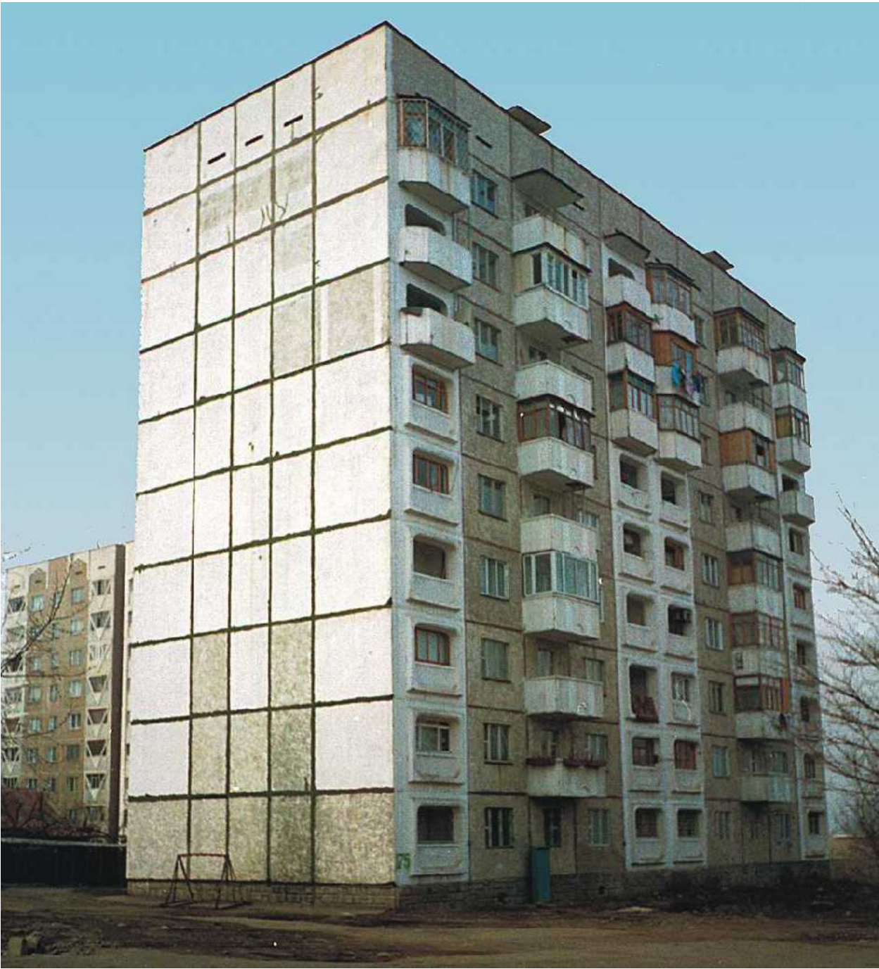
FIGURE 1A: Typical Building
