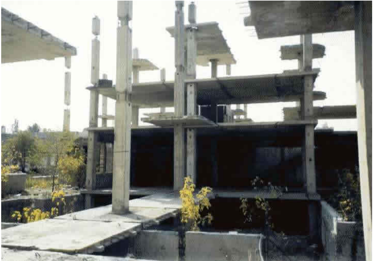
FIGURE 2A: Key Load-Bearing Elements
