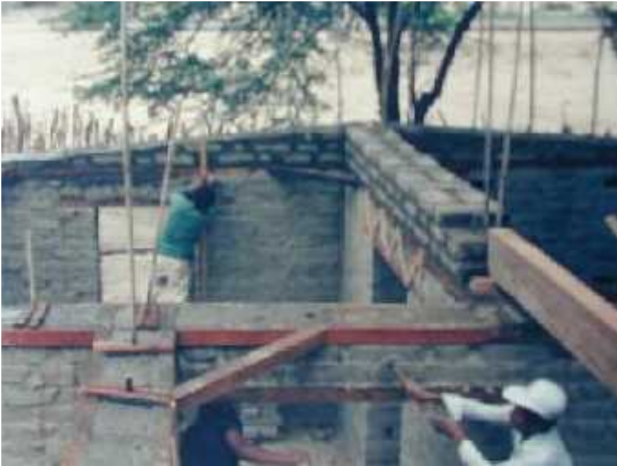
FIGURE 7C: Seismic Strengthening - Construction of Wooden Beams atop the Adobe Walls
