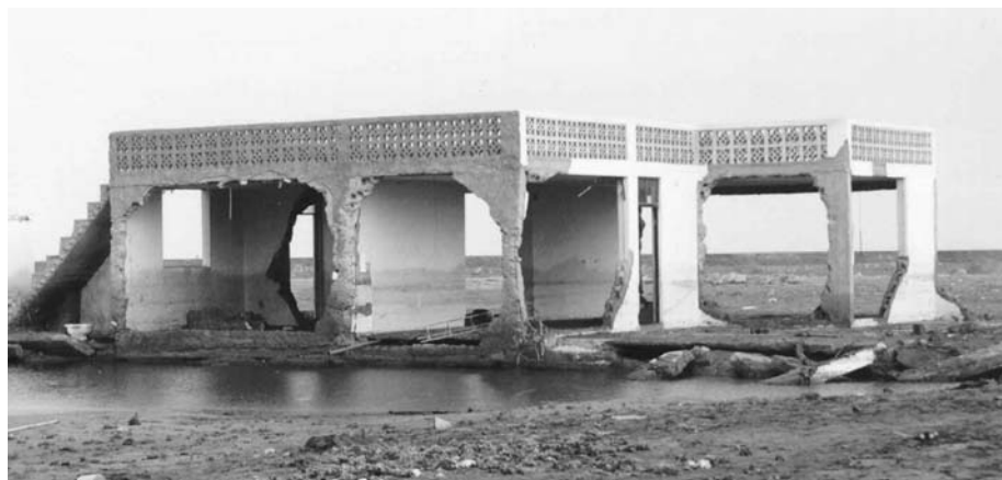
Figure 8 Reinforced column/infilled brick wall structure in the La Punta area. Brick walls perpendicular to wave impact were typically blown out. (photo: Sebastian Araya)
