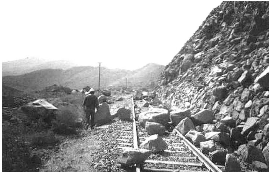
Figure 13 Rock Fall Blocking PeruRail Line. (photo: PeruRail)
