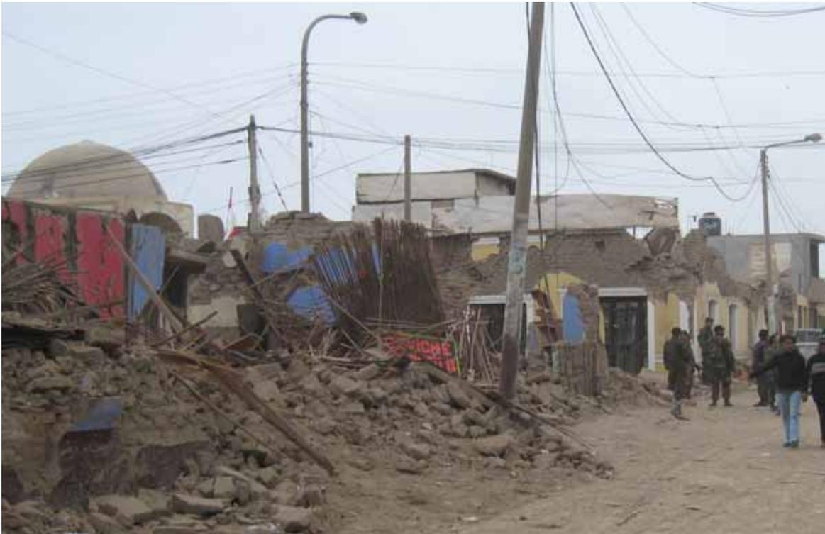
Fig.1 Street in Pisco three days after the earthquake. Most of the adobe houses suffered total collapse. The light blue house at the far right, undamaged, was made of confined masonry.
