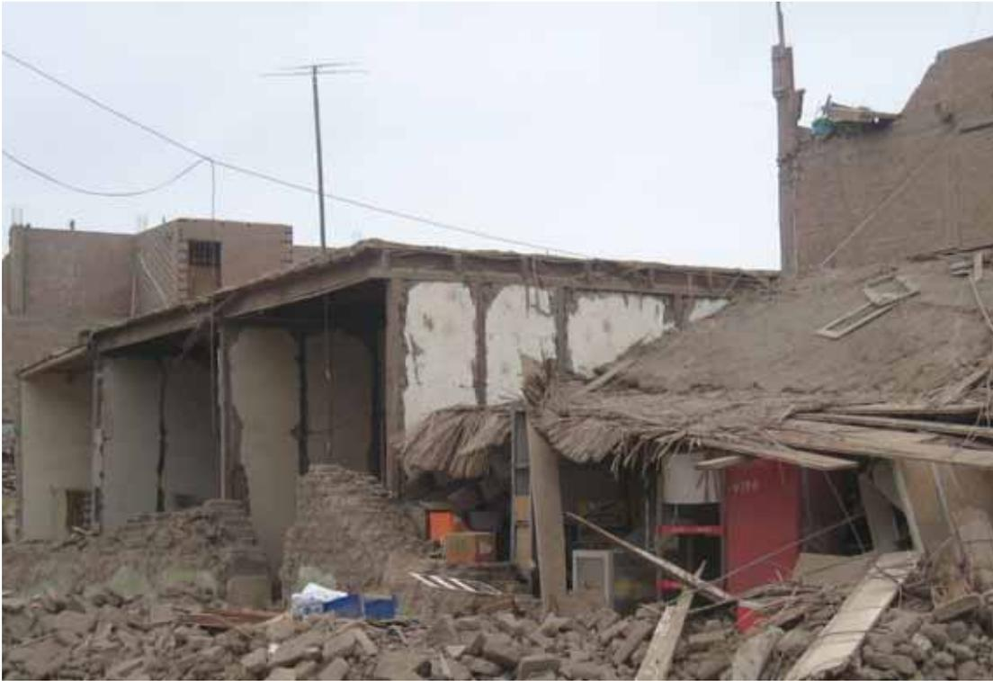
Fig. 2. Two collapsed adobe houses in Pisco. The roof joist of the house on the left are supported on the *quincha* partitions. The roof joists of the house on the right were supported on the façade wall, and thus collapsed with the façade. Notice the undamaged confined masonry house at left, and the collapsed masonry parapet on the house at the back right.
