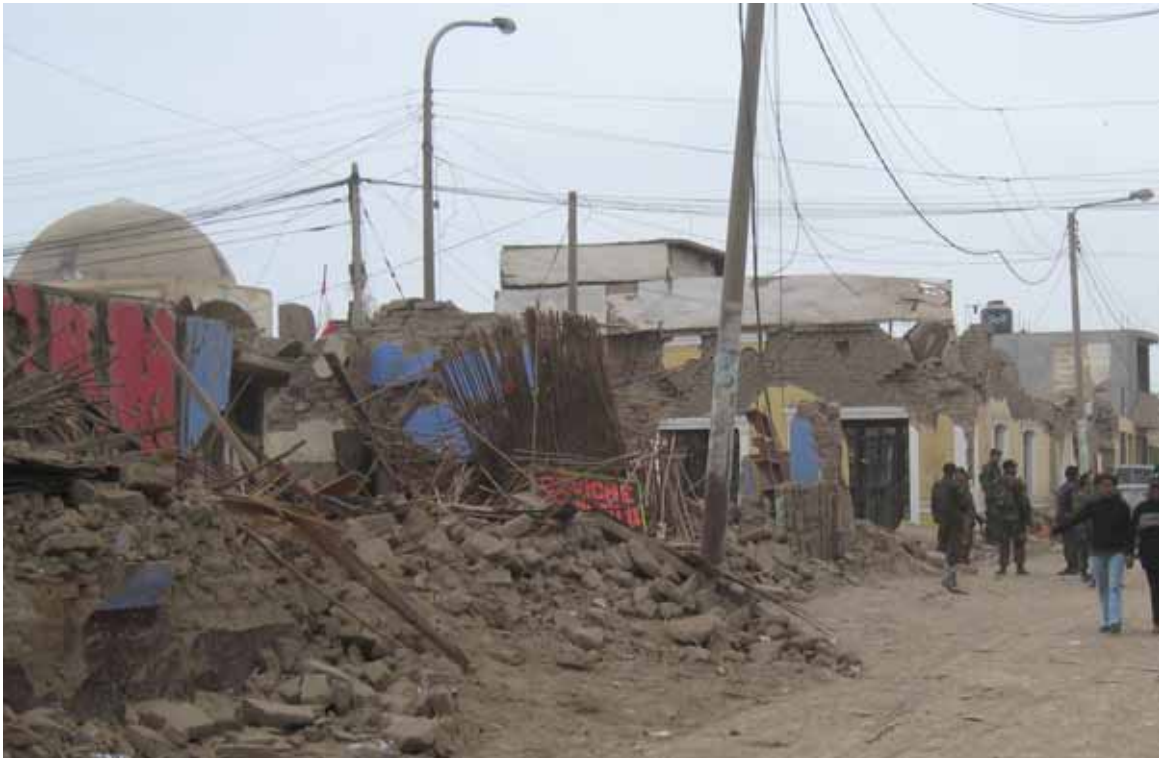
Fig.1 Street in Pisco three days after the earthquake. Most of the adobe houses suffered total collapse. The light blue house at the far right, undamaged, was made of confined masonry.
