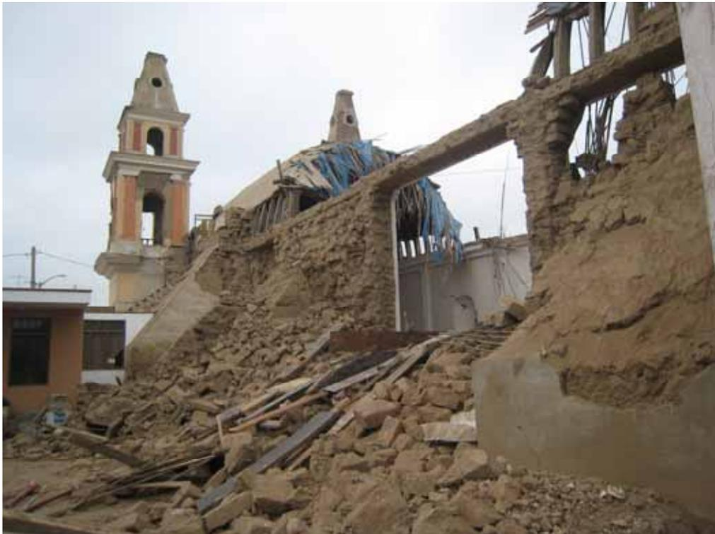
Fig. 4. San Luis Church. The lateral wall and its heavy abutments were practically torn down, presumably by the dynamic thrust of the collapsing vault. The towers are made of *quincha* and suffered little damage.
