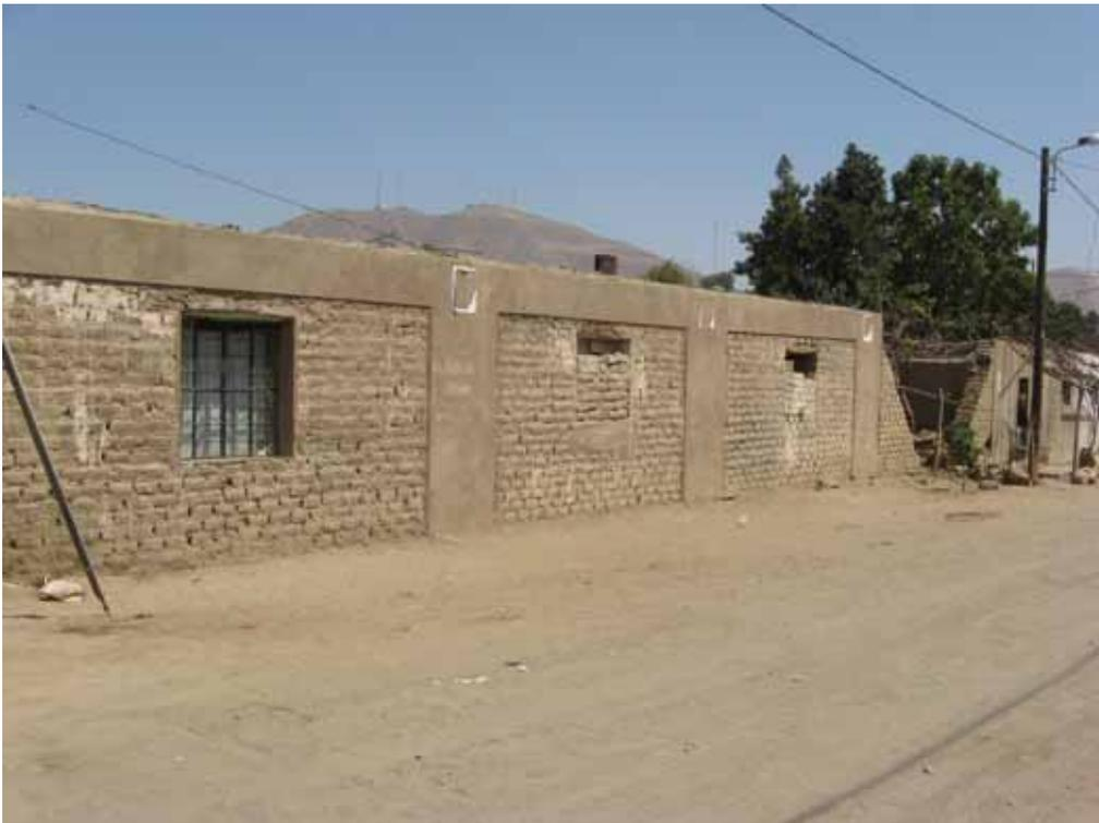
Fig. 3. This undamaged adobe house was reinforced with bands of wire mesh covered with sand-cement mortar. Vertical bands were placed at each wall intersection, and horizontal bands at roof level. Notice the collapsed unreinforced wall at the right.
