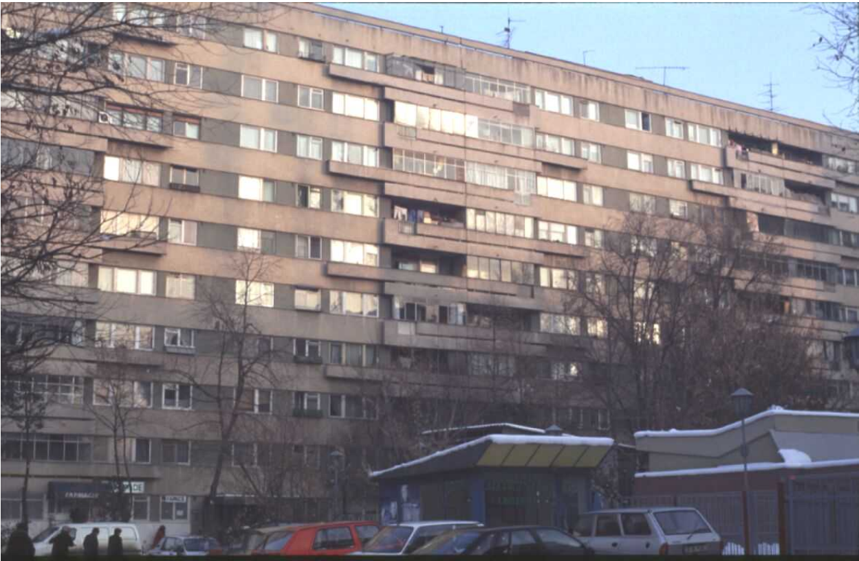
FIGURE 1A: Typical Building
