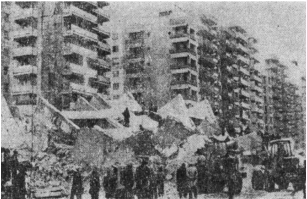
FIGURE 5B: Building Collapse in the 1977 Vrancea Earthquake (OD16 Building)
