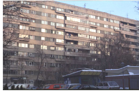
FIGURE 1A: Typical Building
