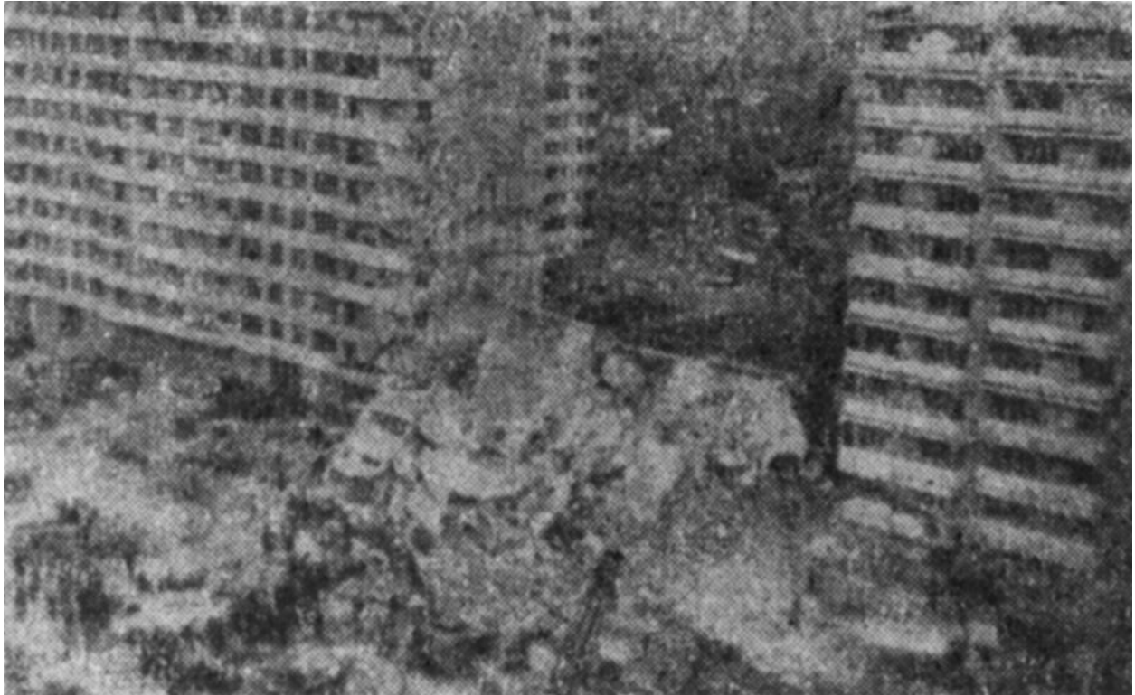
FIGURE 5A: Collapse of OD16 Building in the 1977 Vrancea Earthquake
