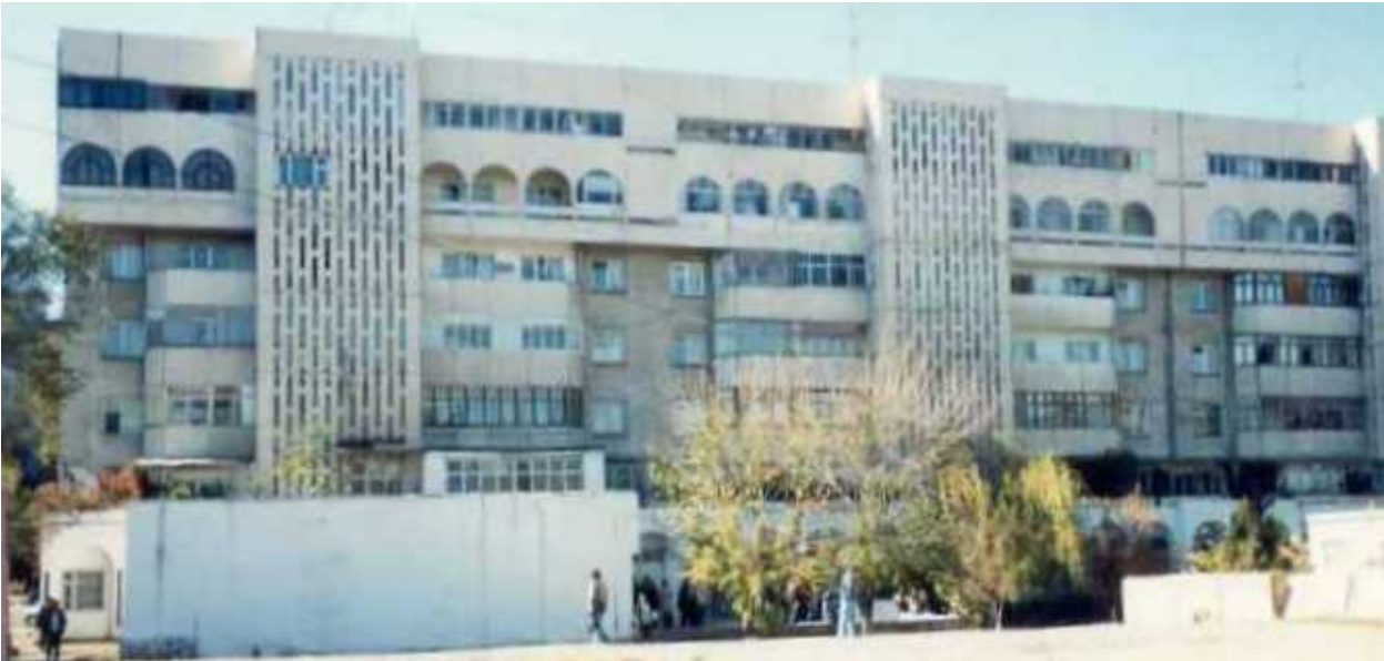
FIGURE 1A: Typical Building - Load-Bearing Masonry Construction (Bishkek, Kyrgyzstan)
