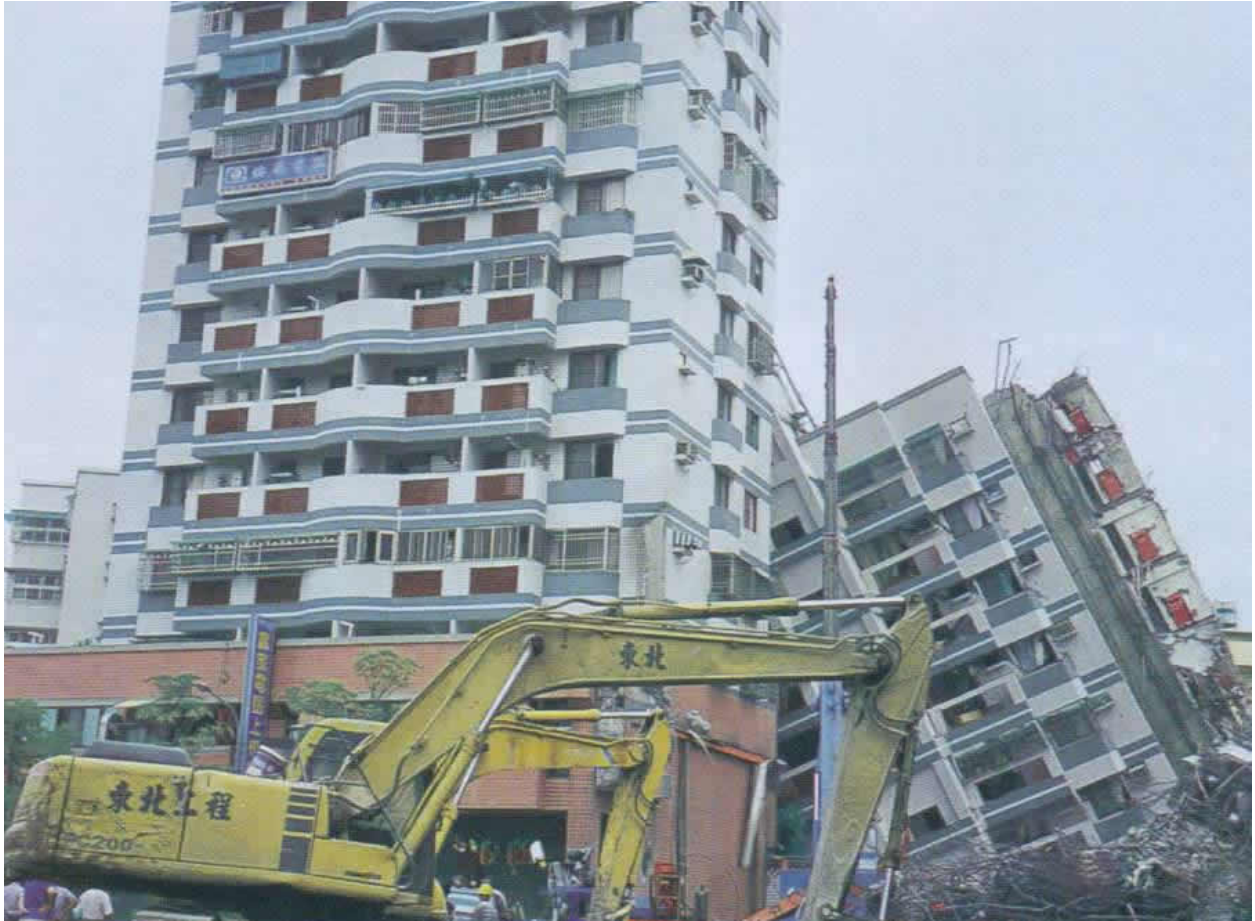
FIGURE 5: A Photograph Illustrating Typical Earthquake Damage
