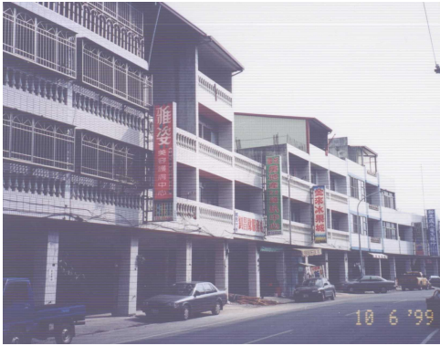
FIGURE 1A: Typical Building
