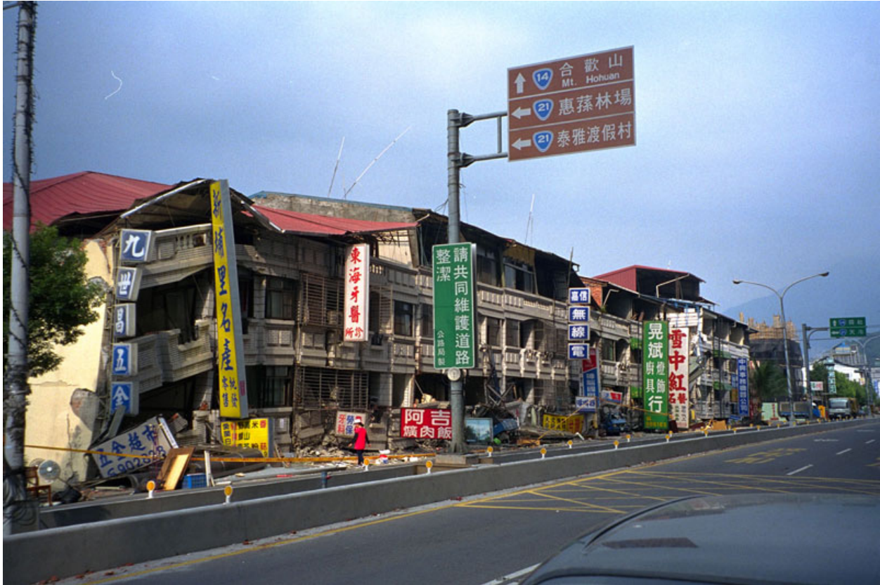
FIGURE 6D: Earthquake Damage - Pancake Collapse of an Entire City Block in the 1999 Chi Chi earthquake (Source: EERI 2001)
