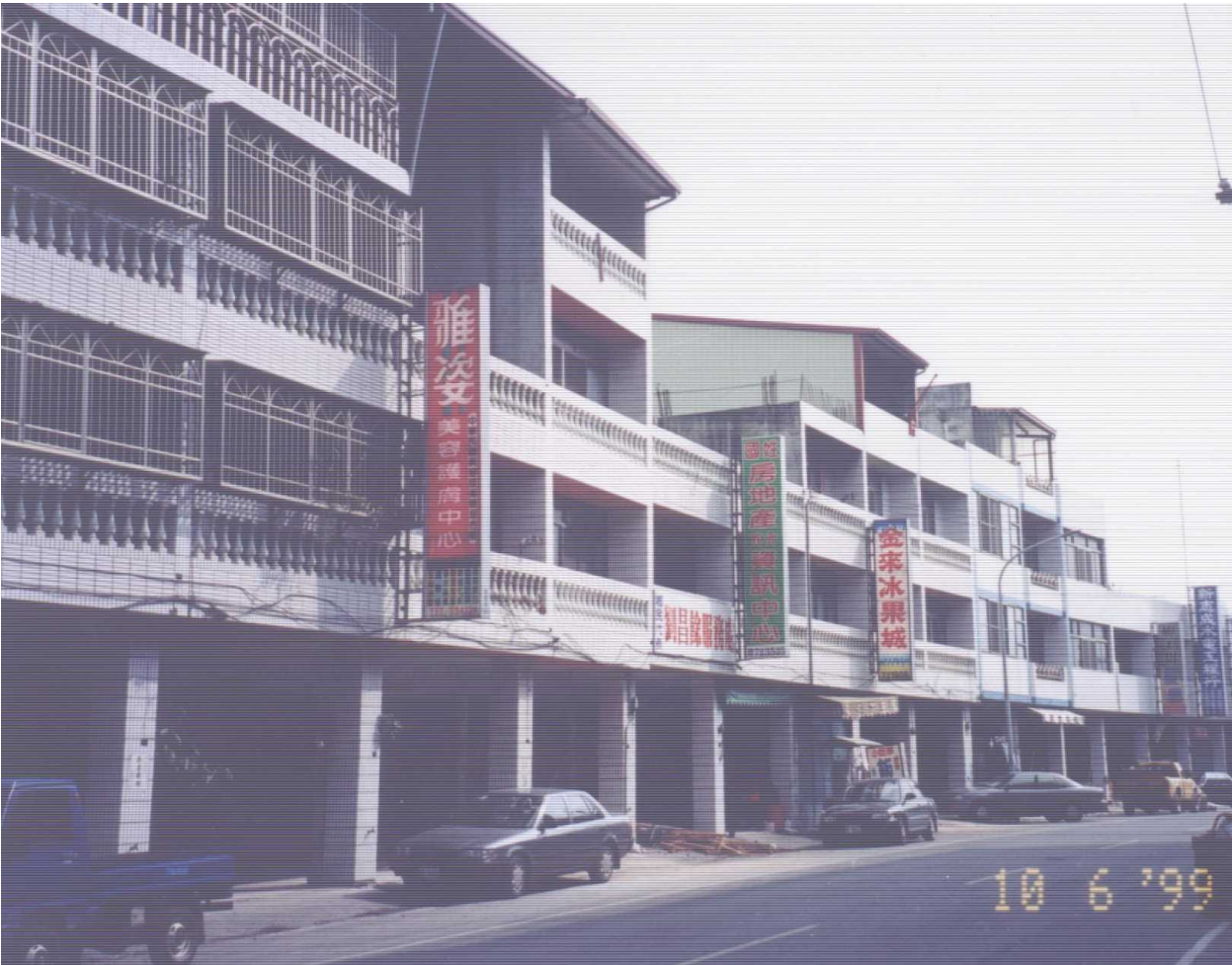
FIGURE 1A: Typical Building
