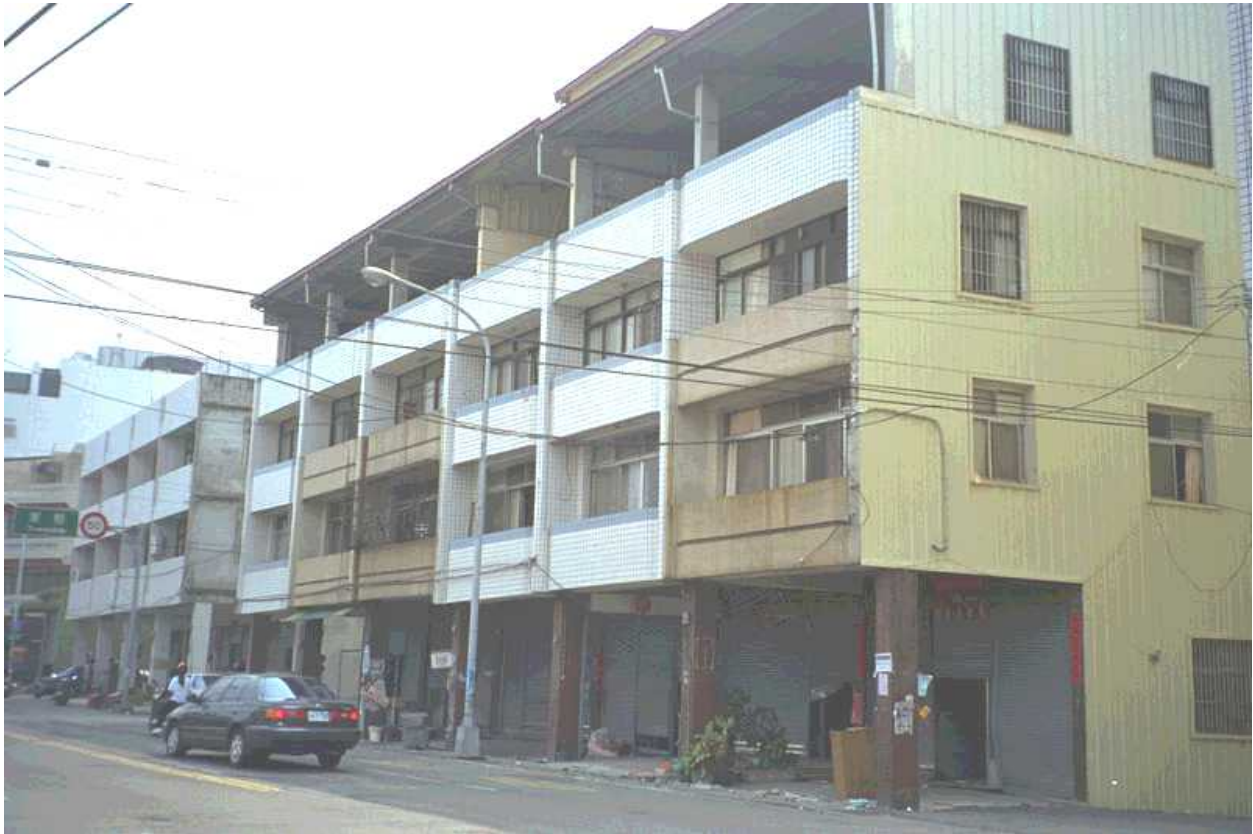
FIGURE 1B: Typical Building (Source: EERI 2001)
