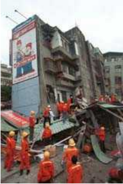
FIGURE 6C: Earthquake Damage - Collapse of a 5-story building in the March 31, 2002 Taipei earthquake
