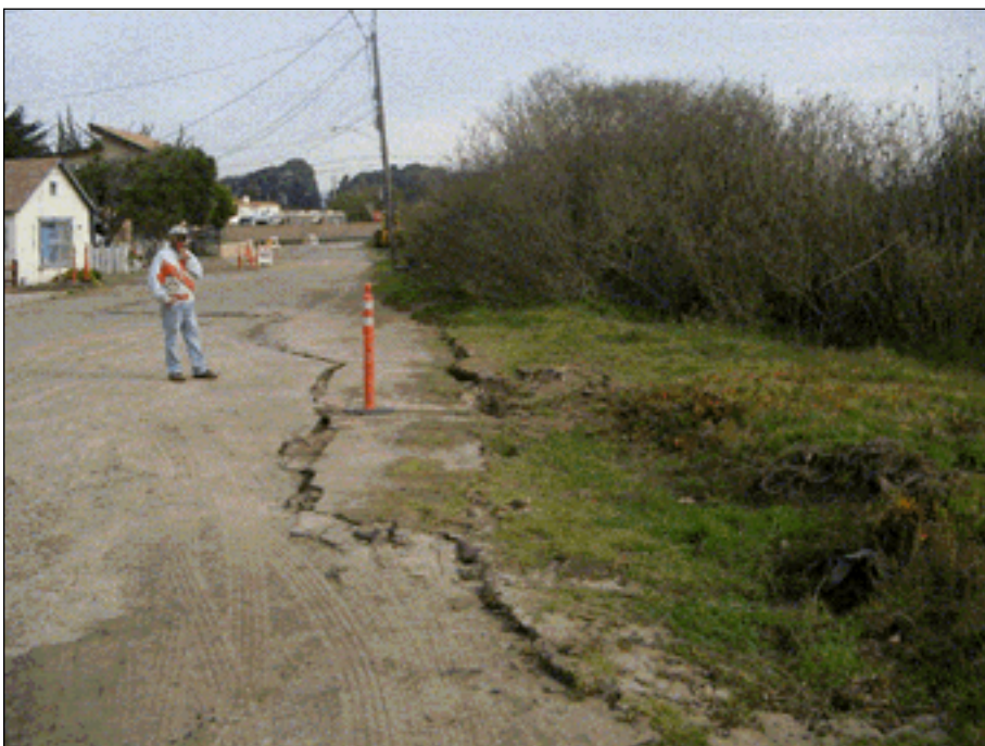
Figure 4. Lateral spread in Oceano (photo Knudsen).
