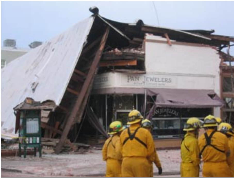
Figure 8. The collapsed Acorn building (photo Marrow).
