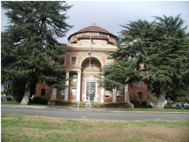
Figure 21. Atascadero City Hall (Picture by Rakesh Goel).
