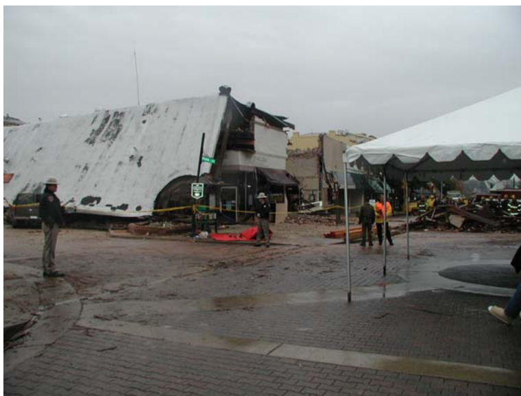
Figure 8. Collapsed Acorn building on the corner of 12 th and Park Streets in downtown Paso Robles (Picture by Rakesh Goel).
