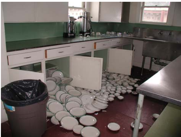
Figure 25. Damage in the kitchen of Atascadero City Hall (Picture by Rakesh Goel).
