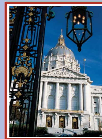
Closed in 1995 after suffering structural damage in the 1989 Loma Prieta earthquake, San Francisco City Hall was renovated, base-isolated, and reopened in 1999 (SFCVB photo by Tom Bross).
