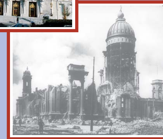
Ruins of San Francisco City Hall dome after 1906 earthquake.
