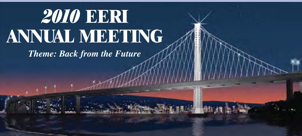
Artist's rendering of the single-tower self-anchored suspension span, the signature architectural feature of the new east span of the San Francisco-Oakland Bay Bridge, to be completed in 2013 (source: Caltrans).
