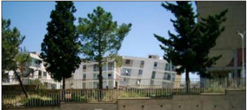
Failure of a multistory residential structure in Algeria (photo courtesy of Michel Sandrin).
