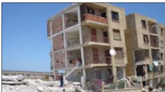
Multistory buildings sustained damage due to failure of columns (photos courtesy of Michel Sandrin).
