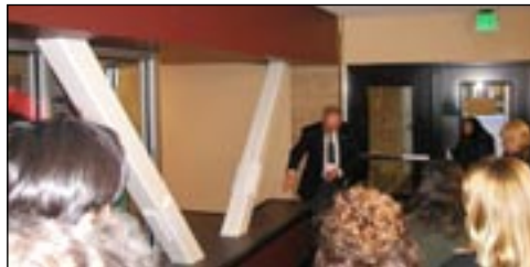
Braced frame in student union building at Portland State University (PSU).
