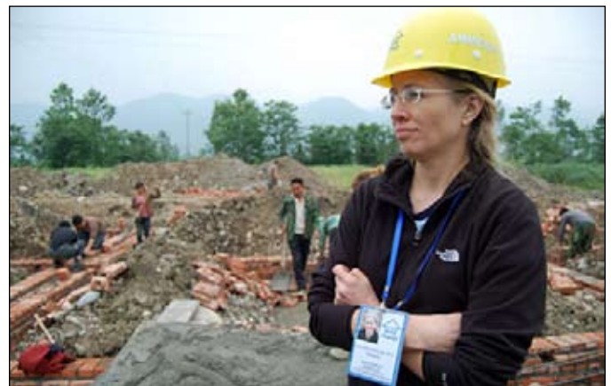
Elizabeth Hausler at a construction site in China (photo: Andrea Hsu/NPR).
