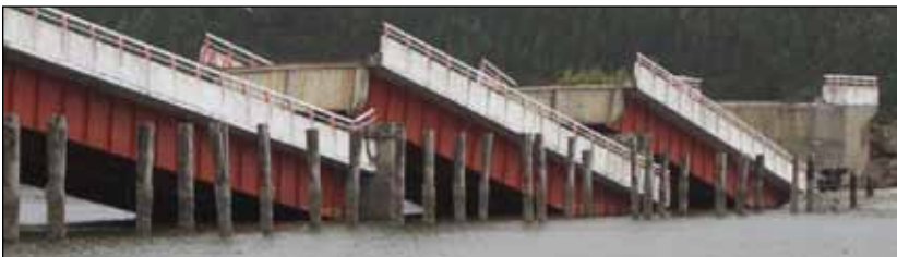
Collapse of 500-ft. bridge in Tubul from strong shaking (photo: Scott Ashford).
