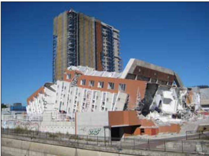
Overturned building in Concepción (photo: Guillermo Franco).
