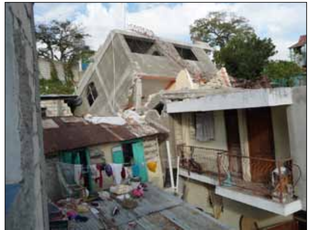
Damage in Jacmel (photo: Martin Hammer).
