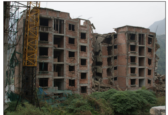
In the old town of Beichuan, a collapsed masonry apartment building was under construction at the time of the earthquake. The entire town has been abandoned and turned into a memorial.
