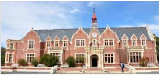
Figure 19. Ivey Hall (a) ▲ at the Lincoln University campus was partially retrofitted prior to the earthquake and performed remarkably well, whereas (b) ► the adjacent unretrofitted Memorial Hall had severe damage at its gable walls (photos: Turner).
