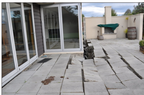
Figure 3. Structures damaged by lateral spreading and post-liquefaction differential settlement. (a) ▲ Residential structure in Spencerville; (b) ► St. Paul's Church in Dallington (photo: Green).
