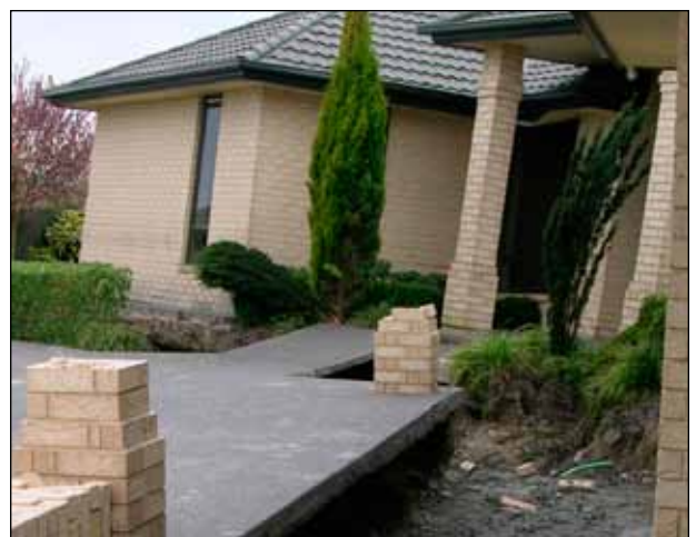
Figure 5. (a) ▲ Large lateral spreading like a rupture passed through the foundation near Courtenay Drive in Kaiapoi. (b) ▼ This house slid more than 1.2 m and tilted significantly (near Courtenay Drive in Kaiapoi) (photos: Lai).
