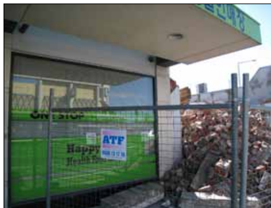
Figure 21. This Asian Supermarket on Riccarton Rd, Christchurch, reopened two weeks after the quake despite damage suffered when the adjacent URM collapsed (photo: Arendt).
