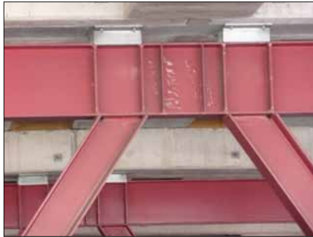
Figure 12. (a) ▲ Yielding in the link beam of an eccentrically braced frame (b) ► and a severely damaged concrete column in a parking garage in downtown Christchurch (photos: Roeder).
