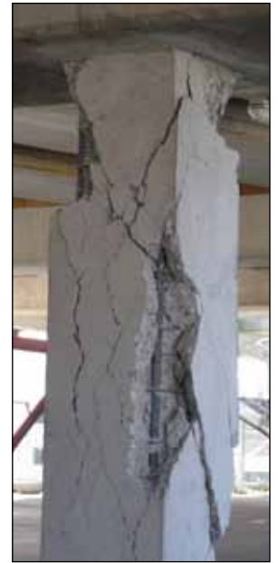
Figure 12. (a) ▲ Yielding in the link beam of an eccentrically braced frame (b) ► and a severely damaged concrete column in a parking garage in downtown Christchurch (photos: Roeder).
