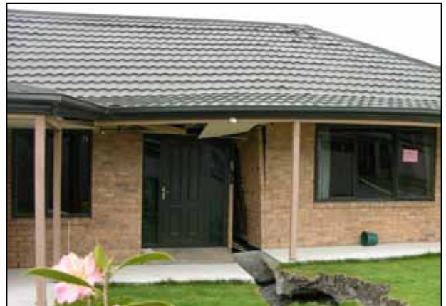
Figure 5. (a) ▲ Large lateral spreading like a rupture passed through the foundation near Courtenay Drive in Kaiapoi. (b) ▼ This house slid more than 1.2 m and tilted significantly (near Courtenay Drive in Kaiapoi) (photos: Lai).
