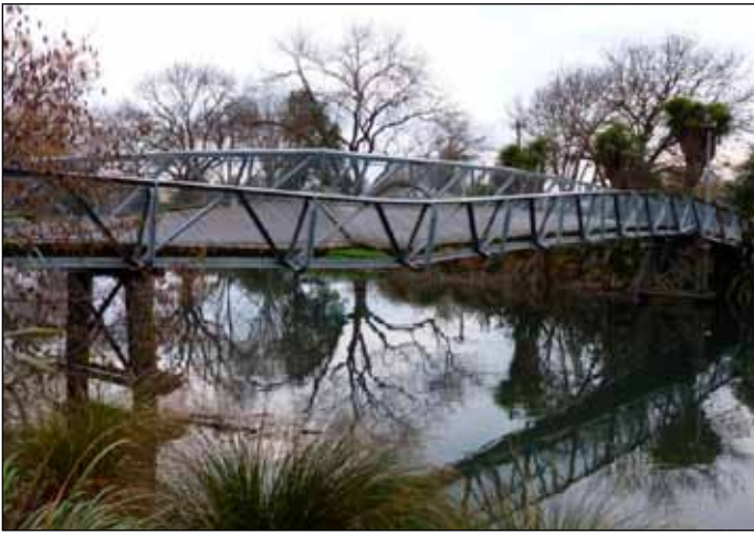
Figure 13. Pedestrian bridge, River Road–Avonside Drive, Christchurch (photo: Bruneau).
