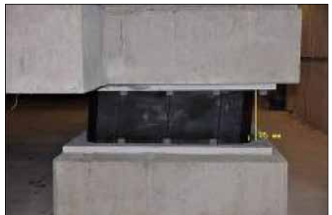
Figure 14. Aspect of the base-isolated hospital building (source: Gavin).
