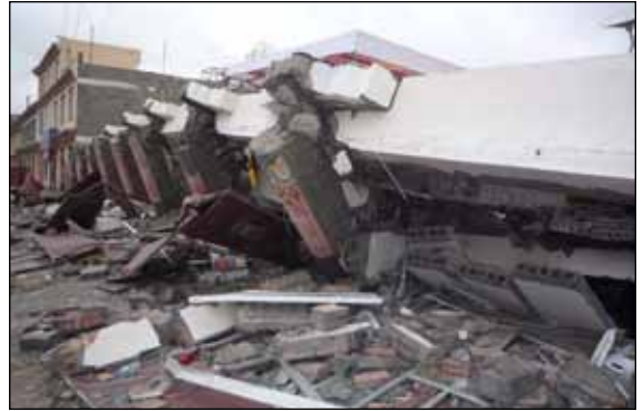
Bottom frame-supported hollow concrete block building collapsed.
