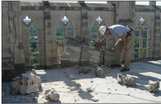
Pinnacle damage at the National Cathedral in Washington, D.C. (photo: Nat'l Cathedral).
