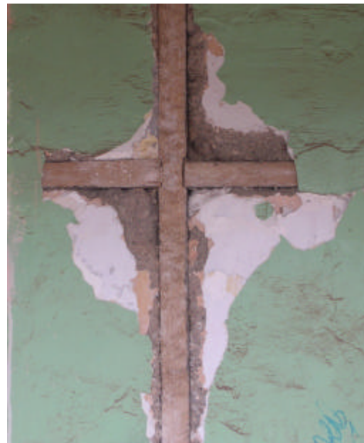
Connection between wooden elements
