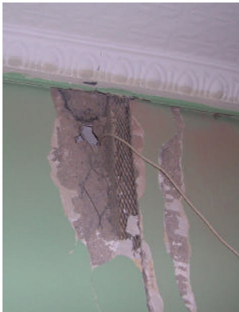
Wire mesh reinforcement
