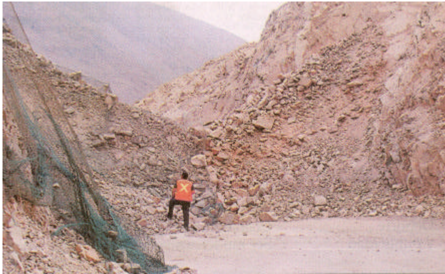
Figure 8 – Landslide at La Paragua, Highway 1 between Tocopilla and Iquique (20 km from Tocopilla).
