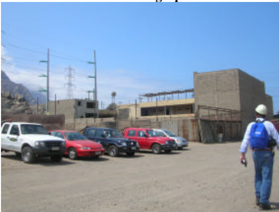
View of some buildings near the accelerograph location on rock in Tocopilla.
