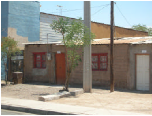
a). House made of adobe in Sierra Gorda
