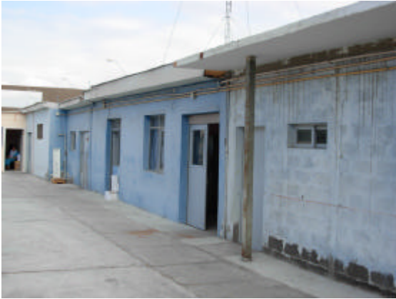
Accelerograph location in the Mejillones Health Center.
