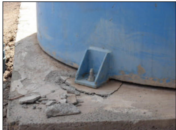
Figure 13 - Damage to filter tank at Baquedano
