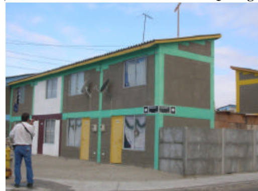
d) Confined masonry house in Mejillones
