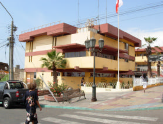
View of the Gobernacion buildings in Tocopilla where the accelerograph is located
