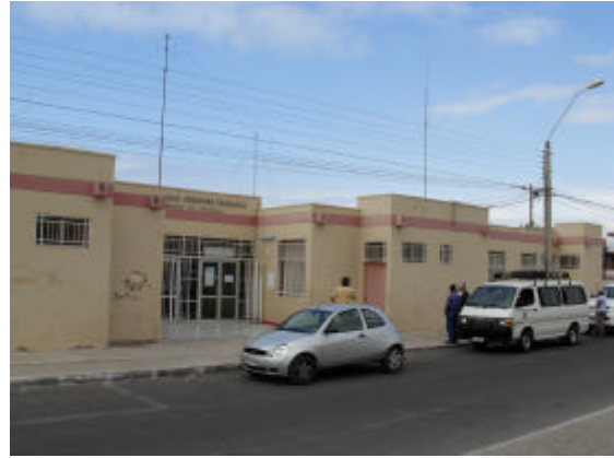
View of undamaged health center in Mejillones where the accelerograph is located.
