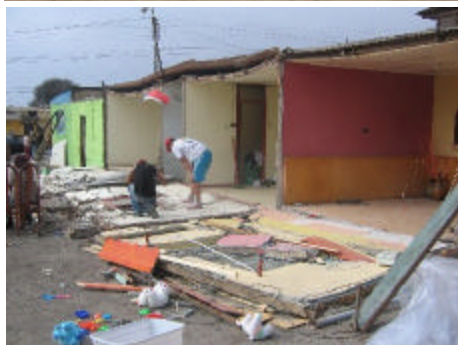
Figure 12. Observed damage: (a) Adobe house in Maria Elena, (b) Wooden frame with adobe infill in Baquedano, (c) Self-construction wooden frame with low quality concrete infill in Tocopilla and (d) Masonry in Maria Elena.
