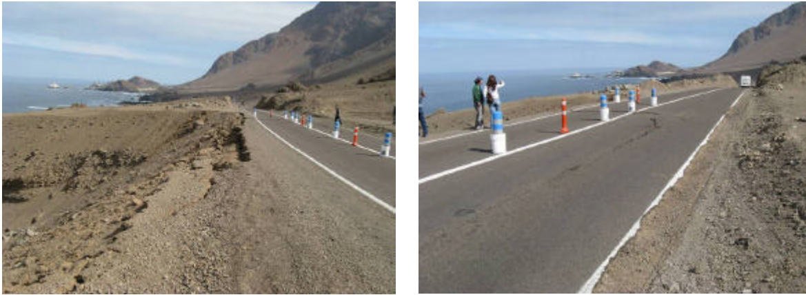
Figure 6 – Landslide and pavement cracking on Highway 1.
