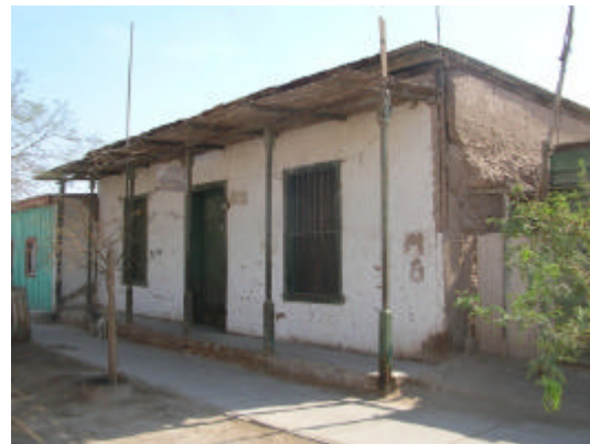
b) Wooden frame with adobe infill in Quillagua.
