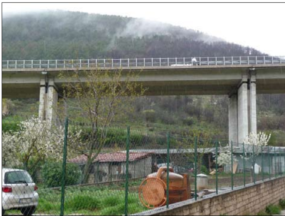
Figure 20. (a) Reinforced concrete highway viaduct that suffered movement of (b, c) bearings and misalignment of columns.
