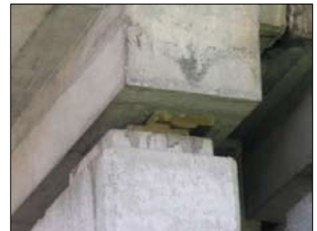
Figure 20. (a) Reinforced concrete highway viaduct that suffered movement of (b, c) bearings and misalignment of columns.
