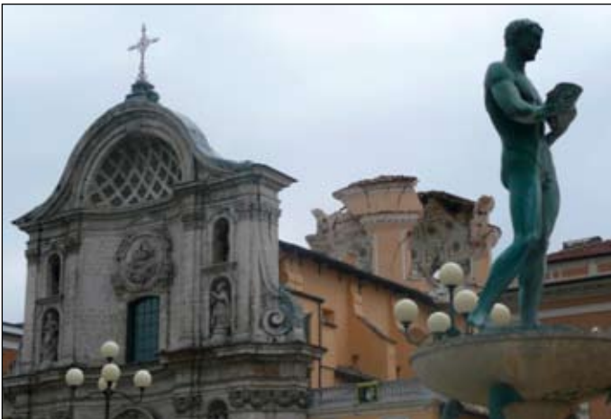
Figure 9. (a) Santa Maria del Suffragio, built after 1703, and (b) Santa Maria di Paganica, both in L'Aquila, lost the roof and cupola.
