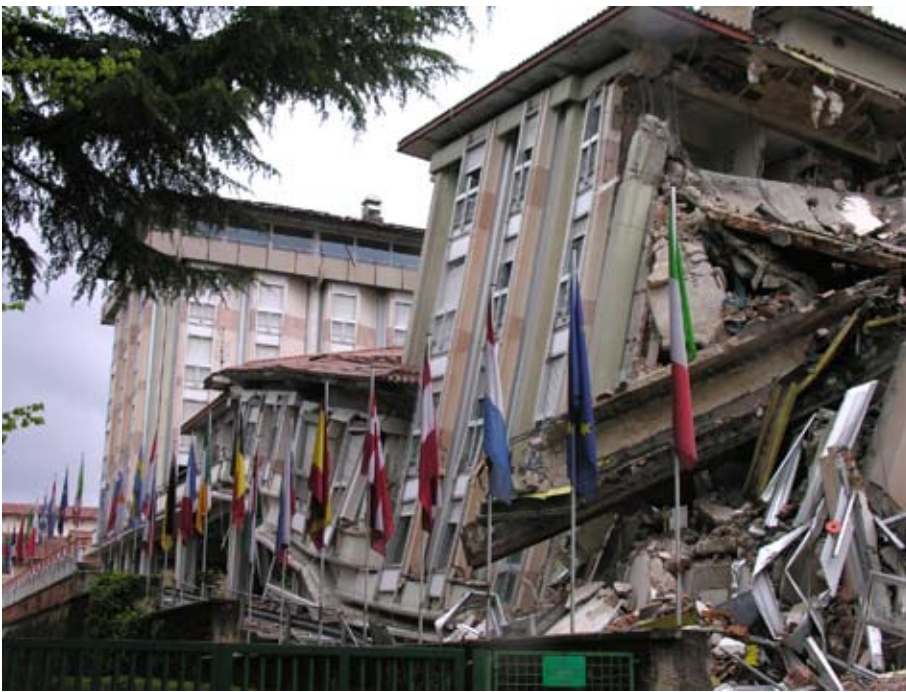
Figure 12. Collapse of part of the Duca D'Abruzzi Hotel caused by a soft-story mechanism. The far part of the building was saved by a seismic separation joint.
