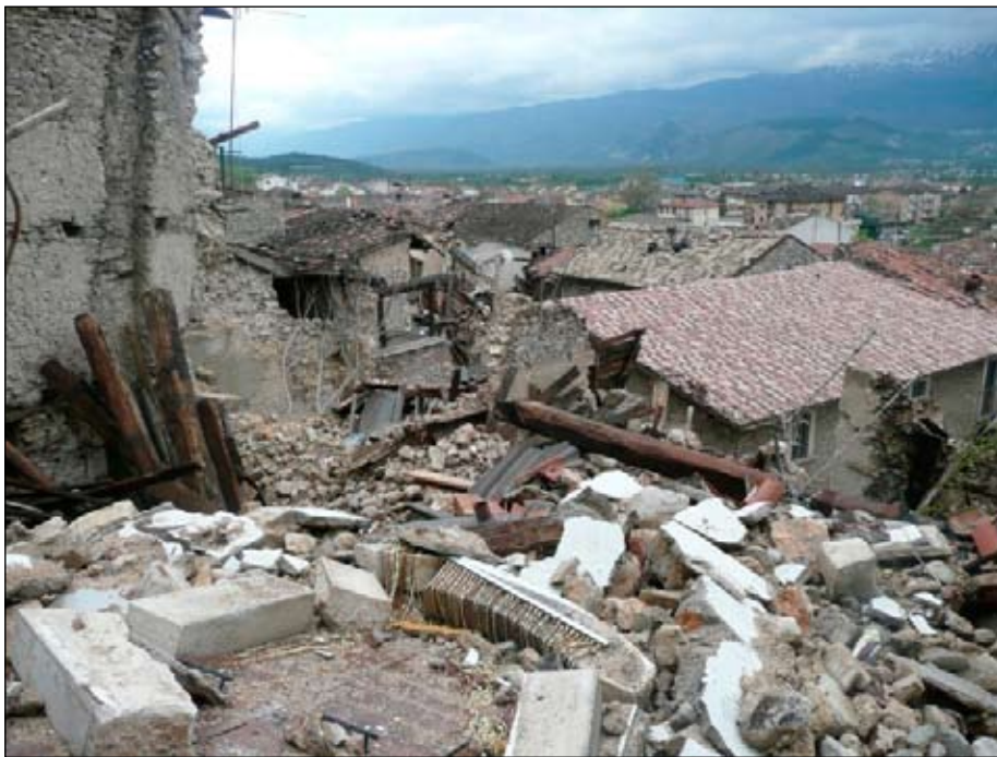
Figure 6. Devastation of poor-quality buildings in Paganica.
