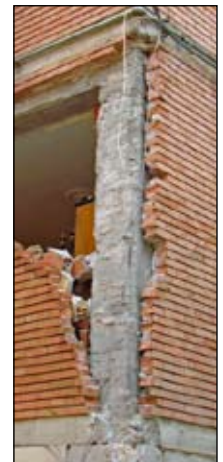
Figure 11a/b. Typical damage to infill walls.
