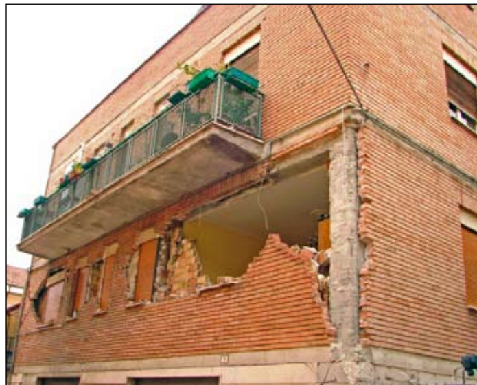
Figure 11a/b. Typical damage to infill walls.
