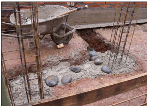
Foundation construction (note tied-column reinforcement cages extending from the foundation)
