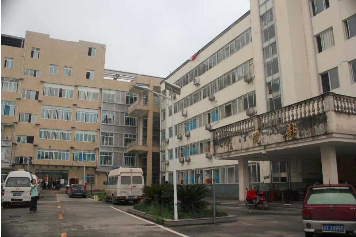
Figure 5. Lushan Hospital. The left building, built after the 2008 Wenchuan earthquake, is base isolated and was fully functional after the April 2013 earthquake. The right building was built before 2008 and is damaged and unoccupied.
