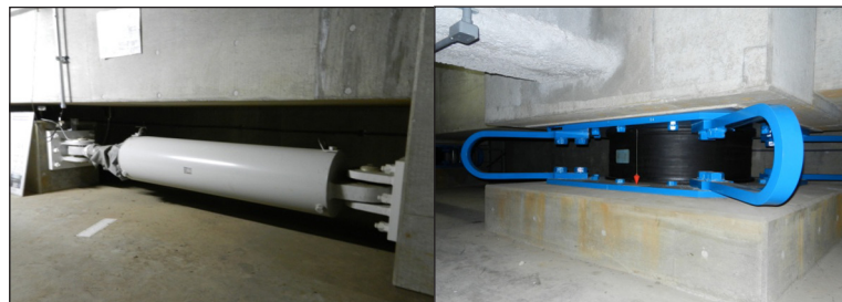
Figure 37. (left) Oil damper, (right) rubber bearing with steel dampers.
