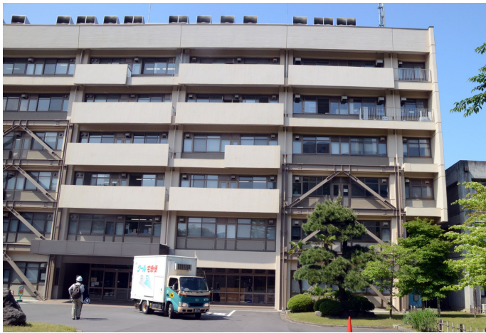
Figure 14. Steel braced frames in Applied Chemistry & Chemical Engineering building.
