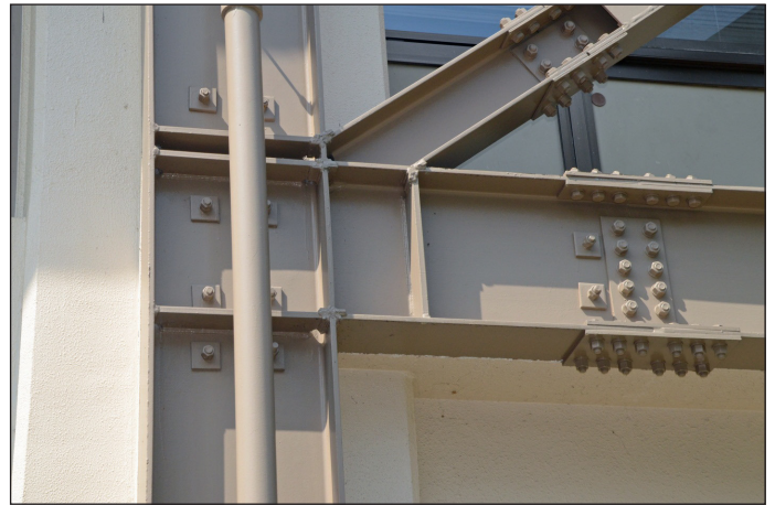
Figure 15. Steel strengthening of concrete building.
