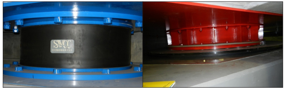
Figure 30. (left) Rubber isolation bearing, (right) sliding isolation bearing.
