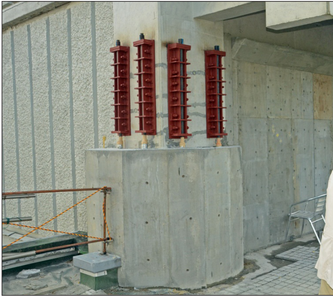
Figure 10. Temporary column repairs with adjacent new concrete walls.
