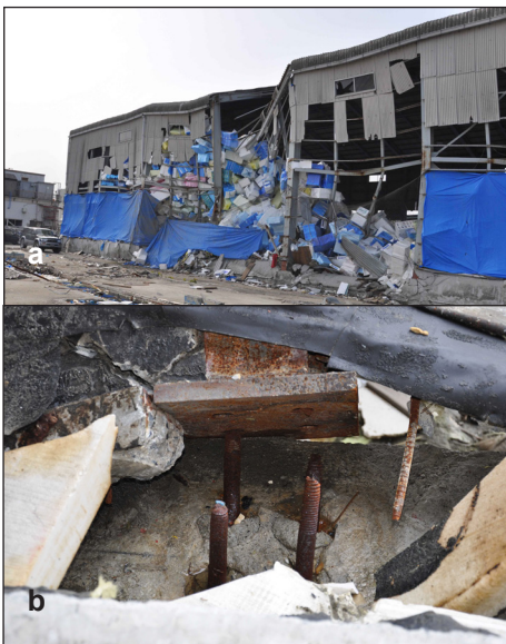
Figure 24. Typical failures resulting from tsunami action in Onagawa and Ishinomaki: (a) deep column twisting (ramming), (b) tensile fracture of steel rods (exposed base plates), (c) base plate cracking, (d) pile foundation failure in toppled steel building.
