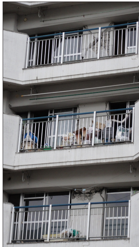
Figure 6. Failure modes for shear panel include diagonal cracking, bond/anchorage slip of vertical reinforcement, and sliding at the top of the panel.
