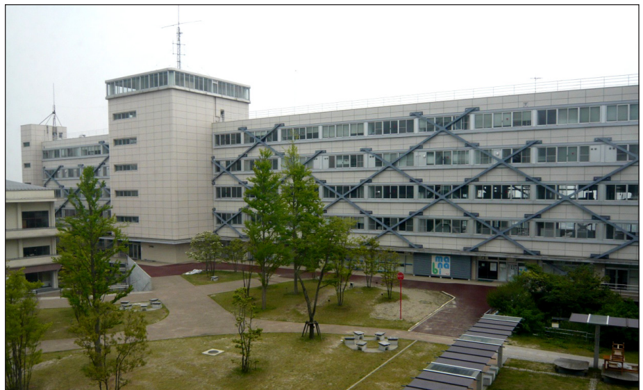
Figure 43. Tohoku Institute of Technology Building 5 with exterior bracing and interior supplemental damping.
