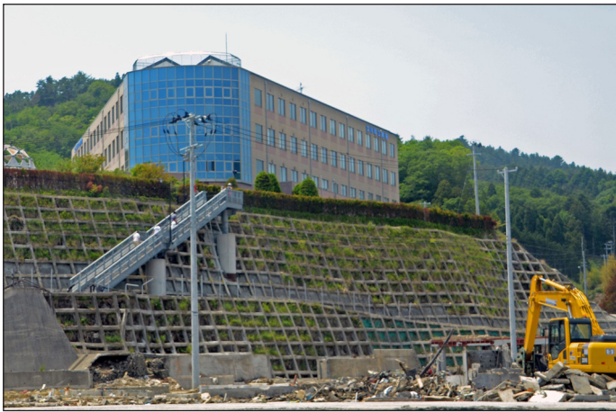
Figure 25. Onagawa hospital on hill above the town.
