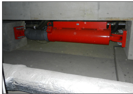
Figure 34. Semi-active damper.
