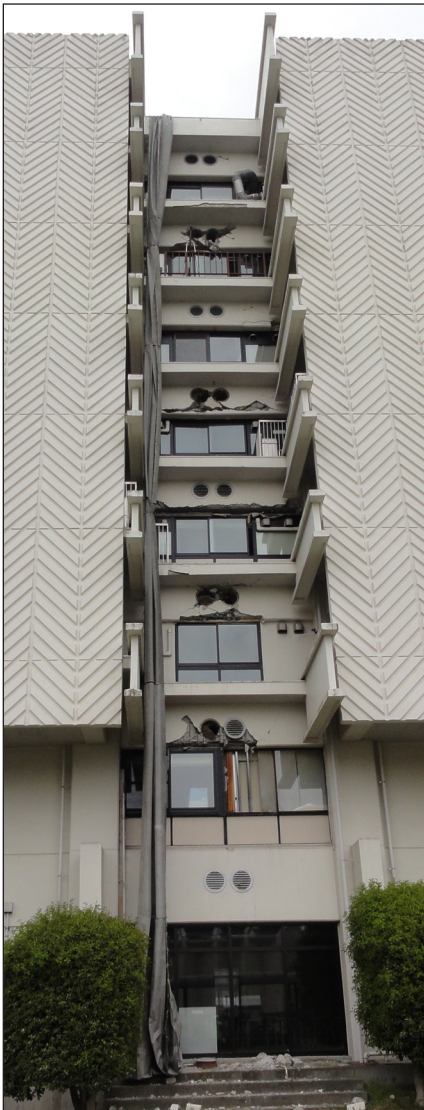
Figure 10. Temporary column repairs with adjacent new concrete walls.
