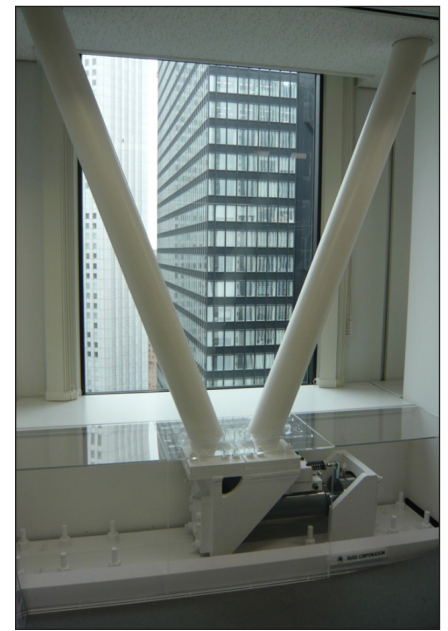
Figure 44. Shinjuku Center Building retrofitted with damper brace.
