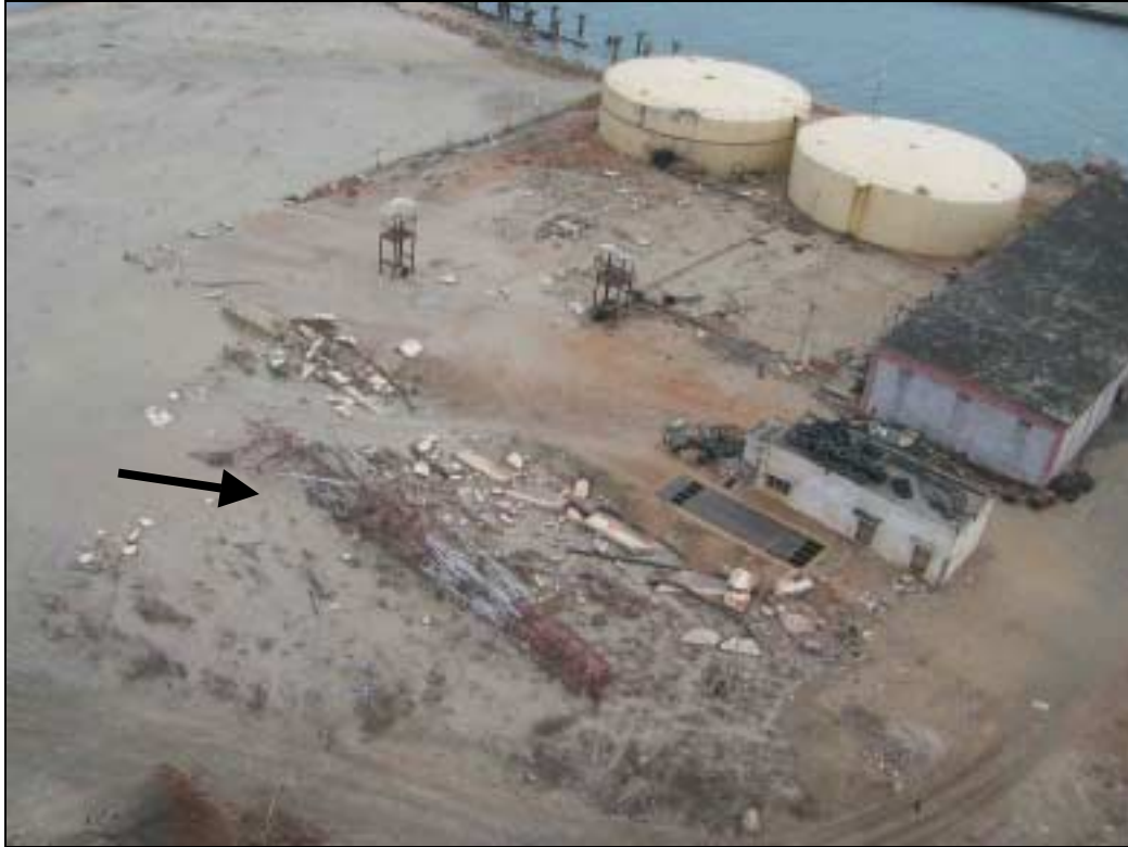
Figure 7. Collapsed telecommunication tower as a result of tsunami (Tang)
