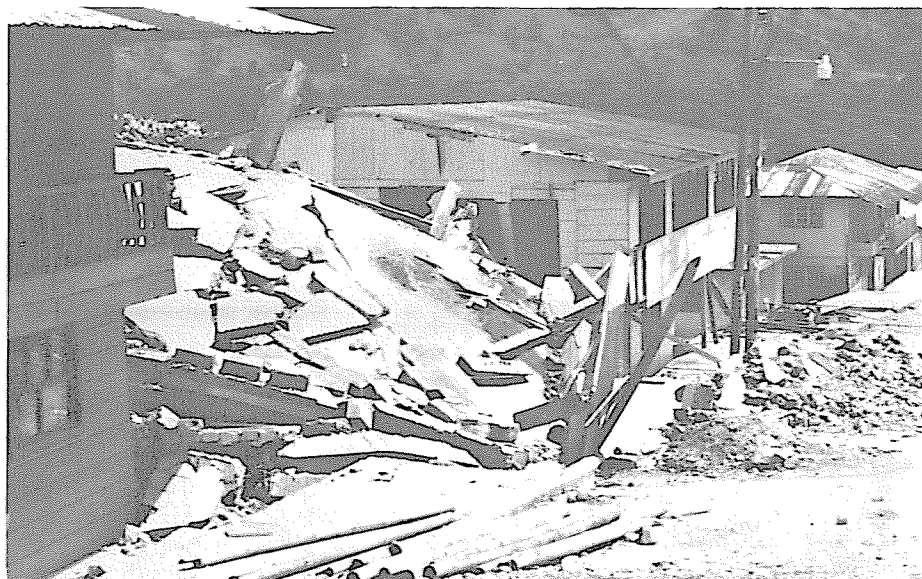
Fig. 4 Collapsed unreinforced masonry structure at Baeza.
