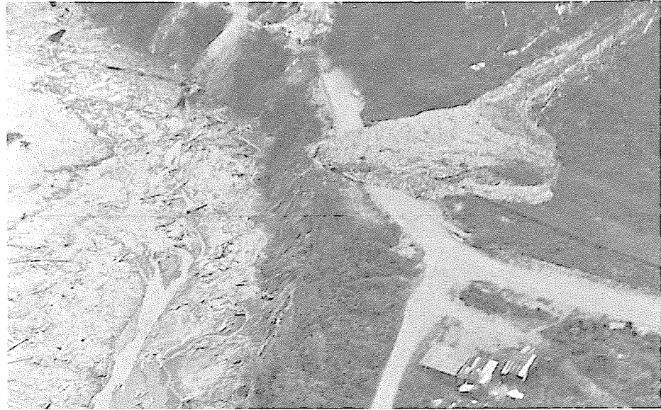
Fig. 2 Trans-Ecuadorian Pipeline damaged by debris flow and erosion. Note oil slick in upper left.
