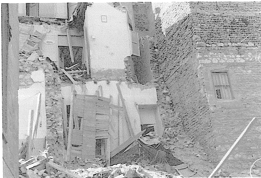
Mixture of stone and mud brick construction
