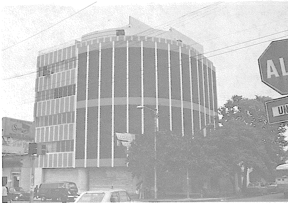
Building No. 16, View Showing Building Configuration
