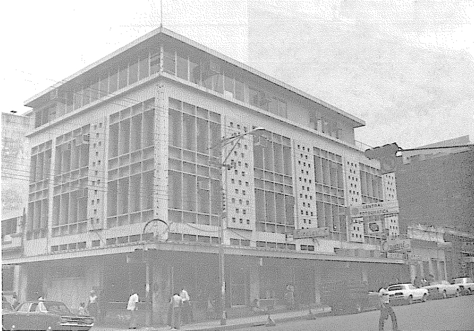
Building No. 13 Ground Level Column Damage
