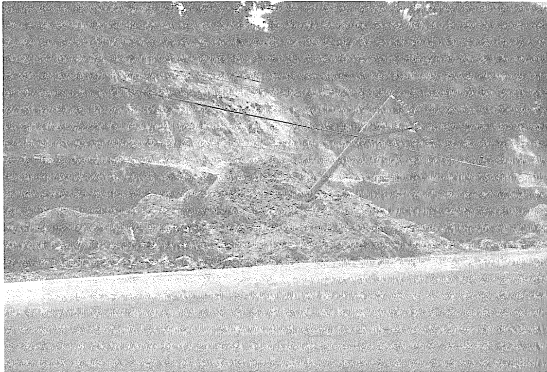
Typical Landslide on Highway
