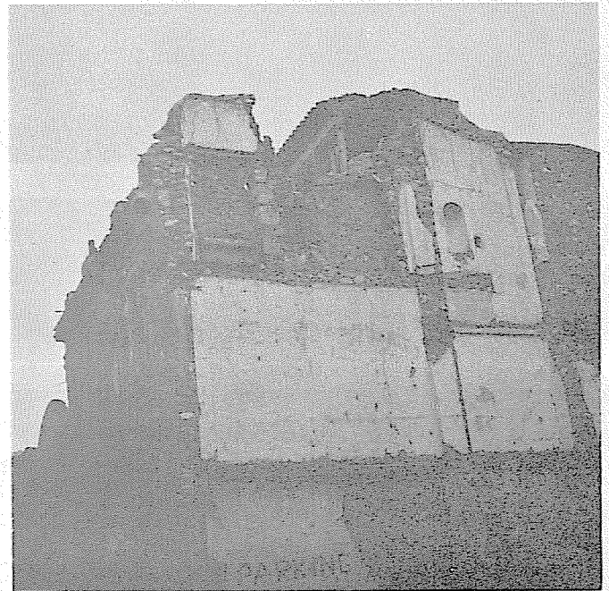
3: Earthquake damage in Athens was only slight.
