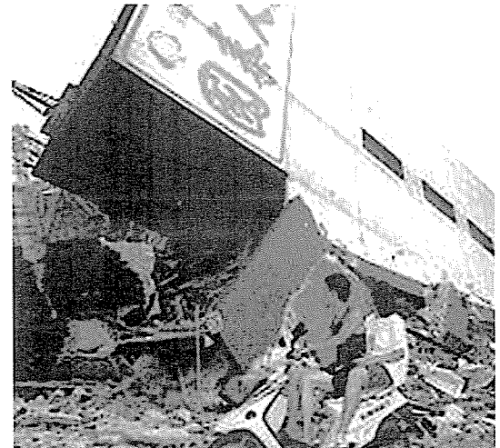
Collapsed building in Nantou County, Taiwan (photo: Agence France-Presse)
