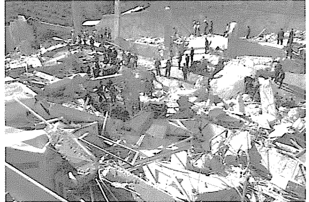
Collapsed factory in northern suburb of Athens, Greece (photo: AP/Dimitri Messinis)
