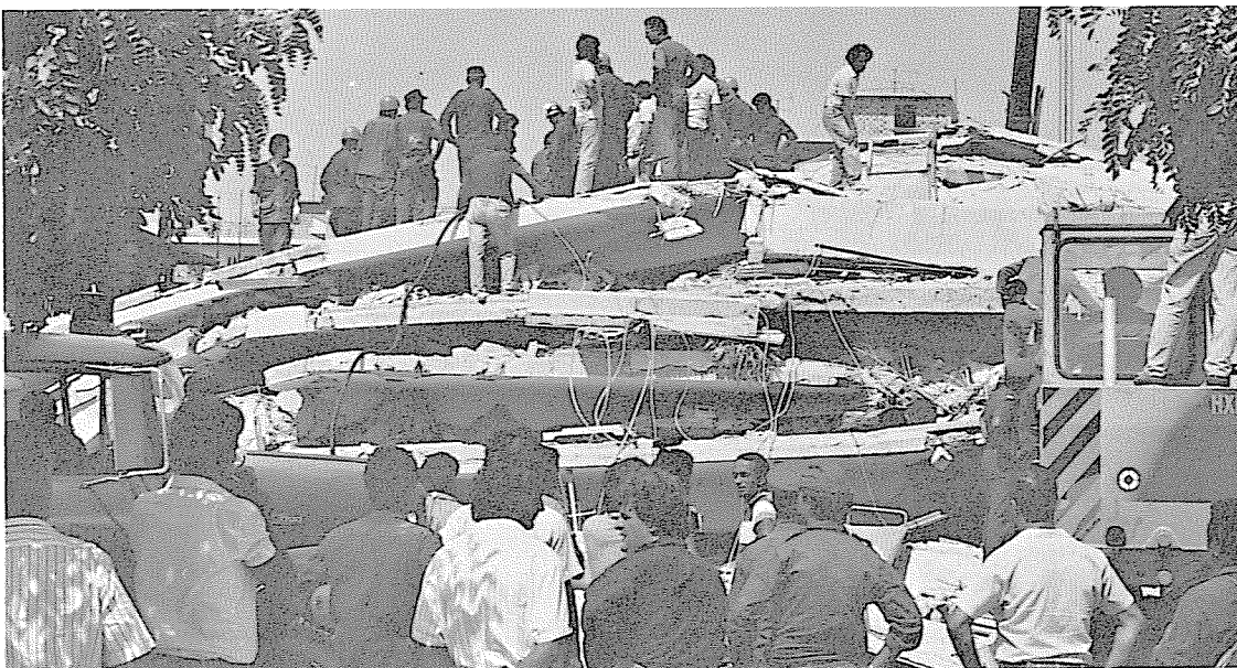
Figure 3. Total collapse of a five-story reinforced concrete apartment building. The partitions are brick walls. Many inhabitants were buried under the debris. The figure shows rescue operations.
