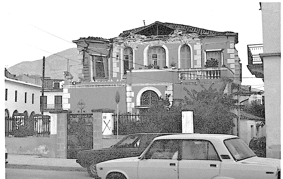
Figure 6. Stone masonry buildings suffered severe damage.
